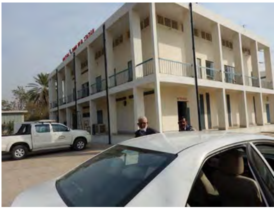
① Control building
