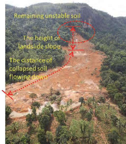
Fig. 10 Landslide at Pahiyangala
