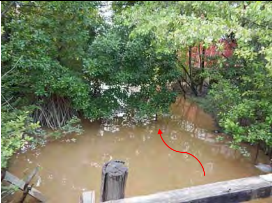
Commerce St. Drainage Channel
