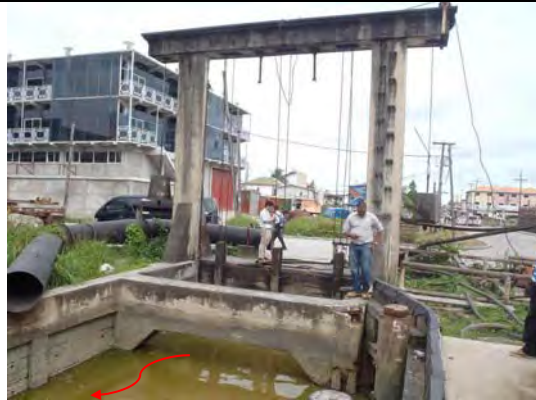
Princess St. Sluice Gate
