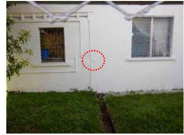
GT7 on Wall of House
