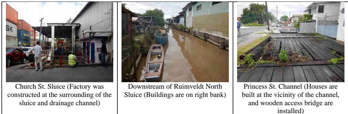
Photo R 2.1.2 Facilities/Buildings along Drainage Channel
