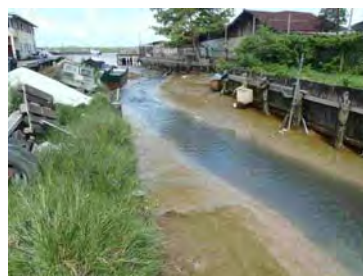
Drainage Channel at Downstream Side of La Penitence South Sluice
