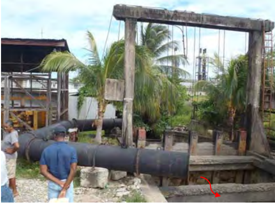
Young St Sluice Gate and Mobile Pump
