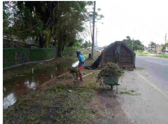
Photo R 2.2.1 Mowing at Drainage Channel
