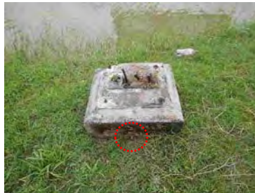
GT13 on Foundation of Former Telecom Facility
