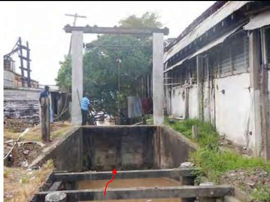
Sussex St. Sluice Gate
