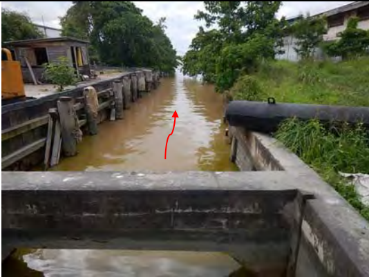
Princess St. Drainage Channel
