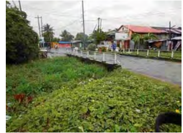
Ruimveldt North Channel
