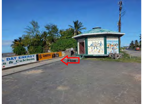
Kitty Pumping Station
