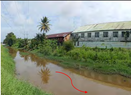
Cummings Drainage Channel
