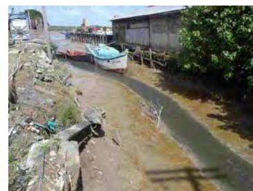
Drainage Channel at Downstream Side of Sussex St. Sluice
