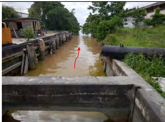
Princess St.排水路
