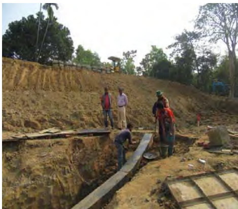
Ph28 Toe Wall construction at up-stream transition end & curing concrete @2017.02.15
