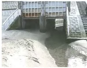
Sediment deposition from apron to box culvert (left) and Vegetation in front of gates (right)
