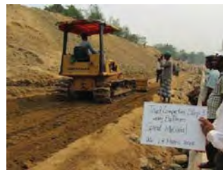
Ph20 & 21. Laying by Bulldozer & Field Density test by sand replacement method
