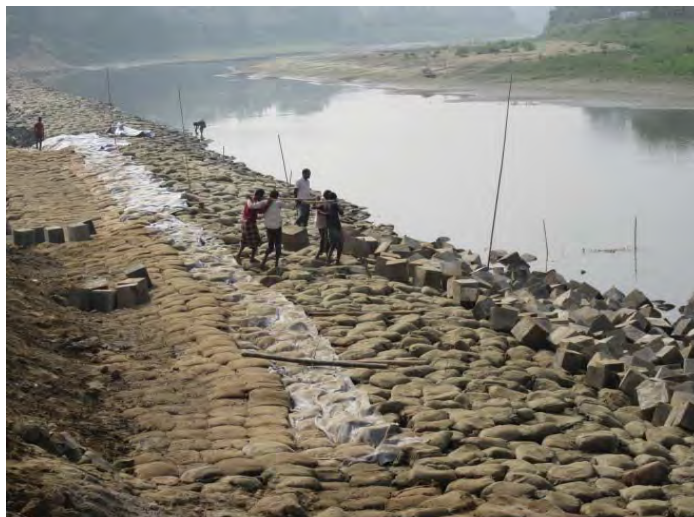
Ph12. One big block (40*40*40cm) is carrying by four (04) nos. labors @2016/02.19
