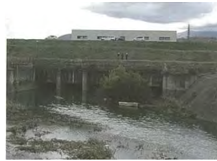
Sediment deposition from apron to box culvert (left) and Vegetation in front of gates (right)
