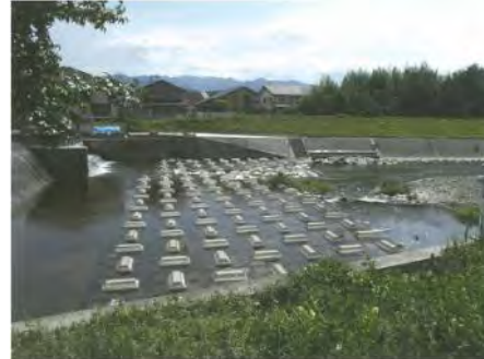
Outflow of foot protection blocks by riverbed degradation
