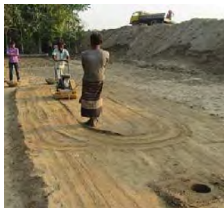
Ph18. Compaction by plate rammer
