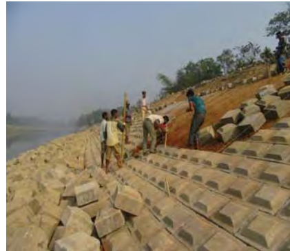
Ph26 & 27 Slope protection works sag in some places are doing correction. @2017.02.01
