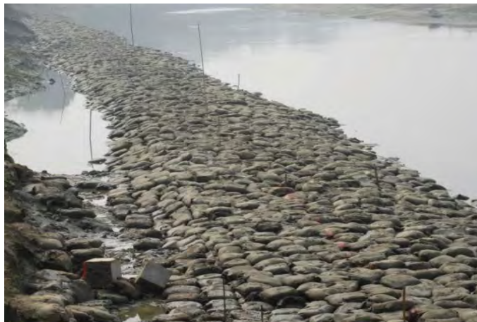
Ph10. Condition of S-C GB mound before dumping of CC blocks and before placing of additional Geo- sheets and local sand filled GB. @2016.02.16
