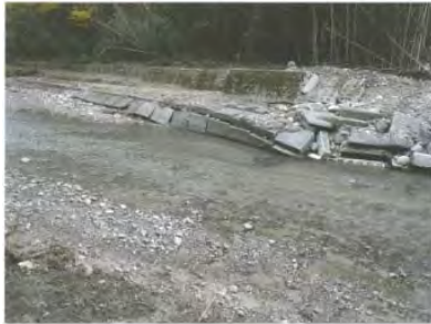
(Left) Deformation of foundation of bank protection by local scoring (Right) Outflow of foot protection blocks by riverbed degradation
