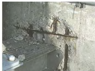
Exposed reinforcing bar due to detachment of concrete (left) and rust of reinforcing bar (right)
