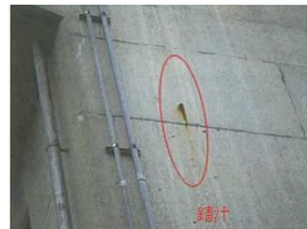
Exposed reinforcing bar due to detachment of concrete (left) and rust of reinforcing bar (right)
