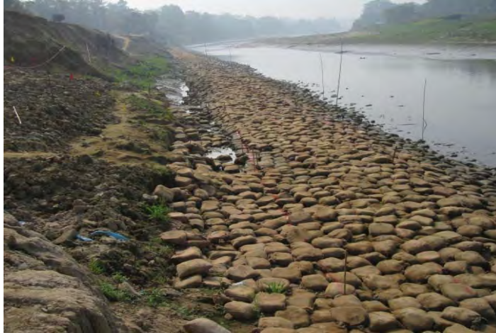
Ph9. Photo taken on 04.02.2016 from the down-stream. Water decreased due to Manu barrage gates closed and water level found 4.20 m(PWD).
