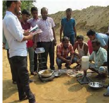
Ph19. Field Density test by sand replacement method
