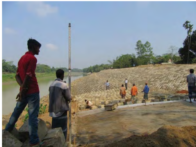
Ph32 Spot levels checked today at up-stream transition area covered Zones (A) and (B) @2017.03.21
