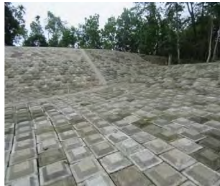
Placing of C.C.blocks at Moulvibazar
