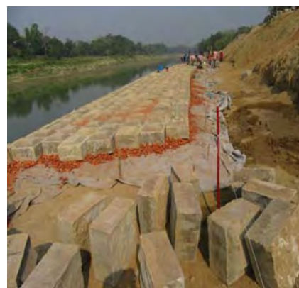
Ph29 View of intermediate berm projected cc blocks laying works from up-stream towards down-stream @2017.02.15
