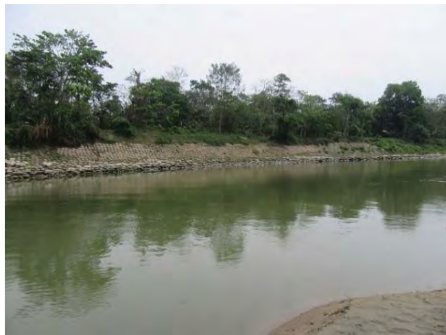
Ph37. Up-stream of PRW temporary protection works. Taken from opposite bank up-stream of grave yards. @2017.03.09
