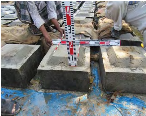
Manufacture of C.C.blocks at Moulvibzar
