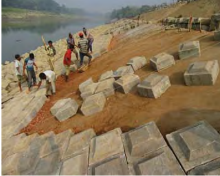
Ph26 & 27 Slope protection works sag in some places are doing correction. @2017.02.01
