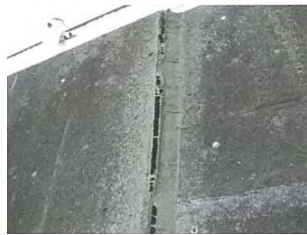
Opening at joint (left) and crack on box culvert (right)
