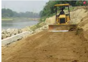
Ph17. Compaction by bulldozer
