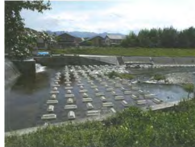
(Left) Deformation of foundation of bank protection by local scoring (Right) Outflow of foot protection blocks by riverbed degradation
