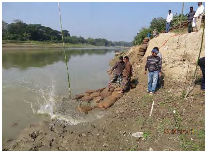
Ph7. On 21 Dec 2015, duping S-C GB started from the down stream
