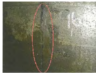
Opening at joint (left) and crack on box culvert (right)
