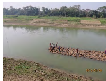
On 8 Jan 2016, ditto from the down & middle stream, 2,390bags dumped
