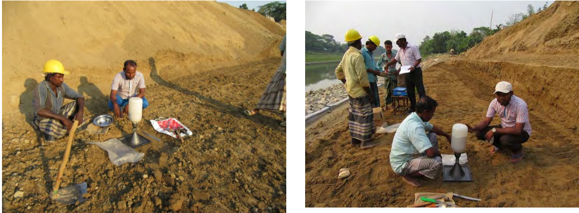
Photo 3.4.4 Field density test (sand replacement method)
