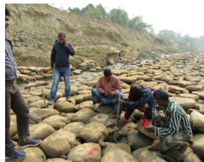
Set formation level and alignment & check remaining works on 16 Jan op6
