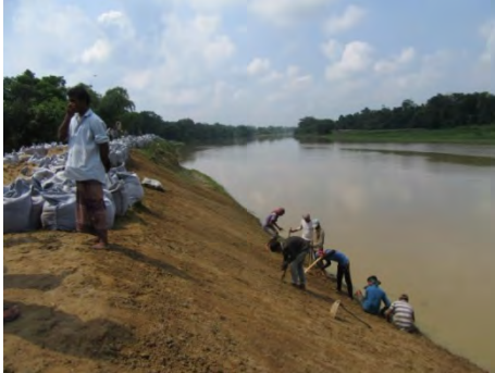
Dressing the surface of earth of slope before laying Geo-sheet on 2016.06.2
