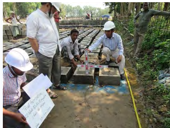
PhD. Checking completed shape of projection part as per design
