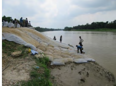
Laying geo-sheet and geo-bag on the slope on 2016.06.02
