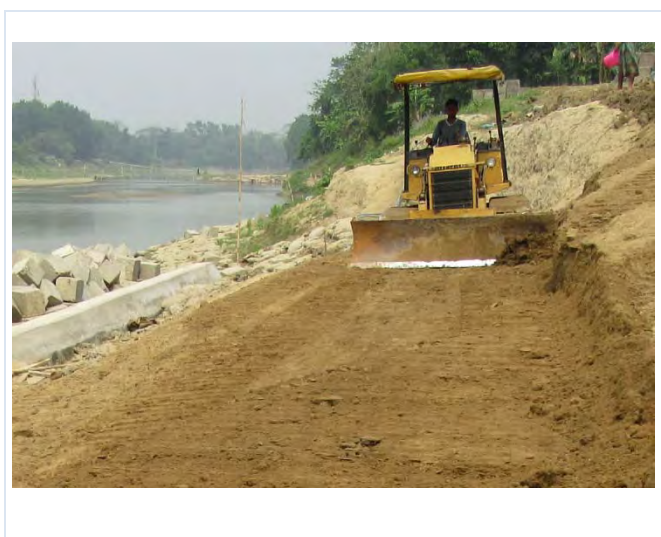
Photo3.4.1 Spreading & compaction by bulldozer
