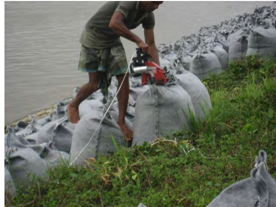
Photo 4.1.1 On-site geo bag sand packing
