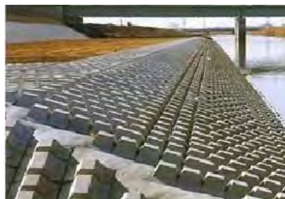
Photo 4.2.2 Example of prefabricated CC-block in Factory and layout on the slope ( Example size: 480mm × 250mm × 250mm (45.7kg))
