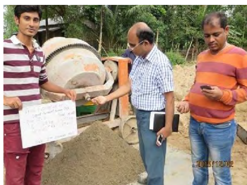
Checking workmanship after mixing sand cement
