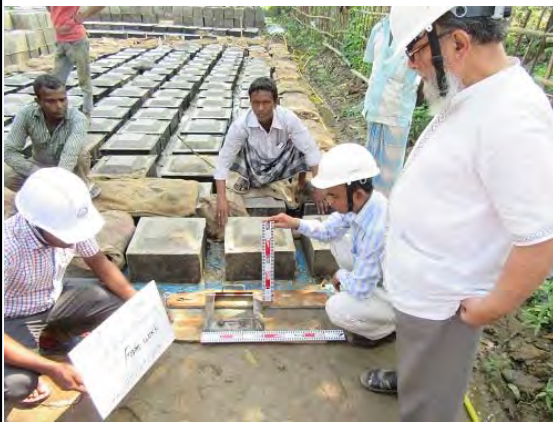
PhA. Checking steel made formwork, with require dimensions
