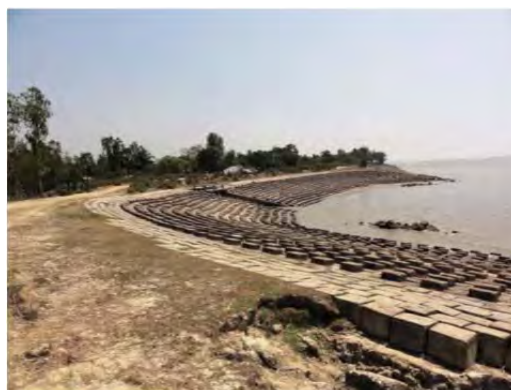
Photo 4.2.1 CC-block on Revetment
