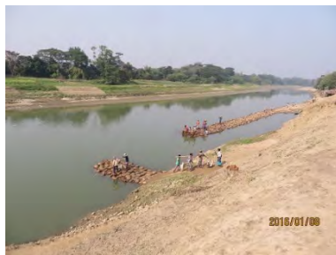
On 8 Jan 2016, ditto from the down & middle stream, 2,390bags dumped
