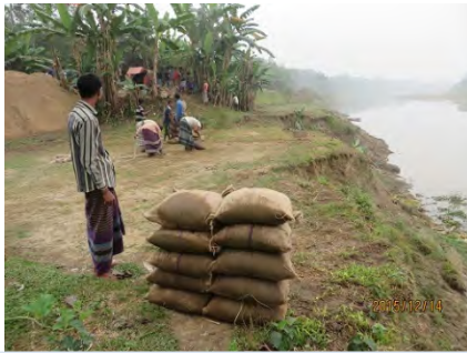
From 14 Dec2015, Start stockpile
