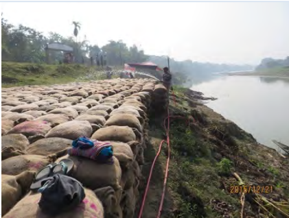
Curing at Yard 2 on 21 Dec 2015
