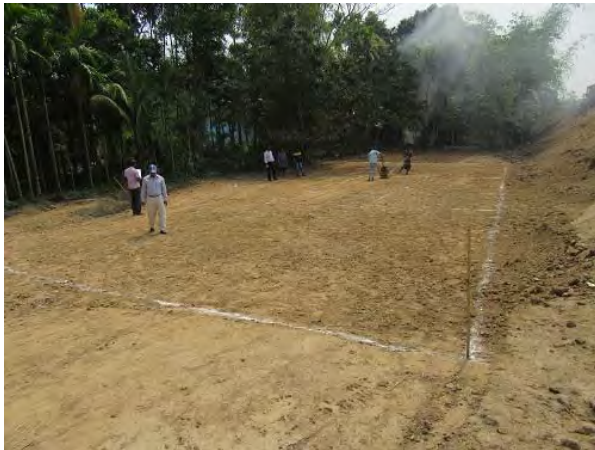
Ph A. Preparation for testing yards (backfilled existing Pond)
