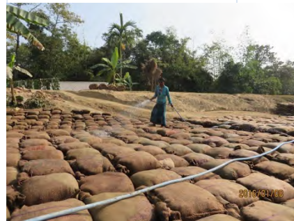
Curing at Yard 1 on 8 Jan 2016
