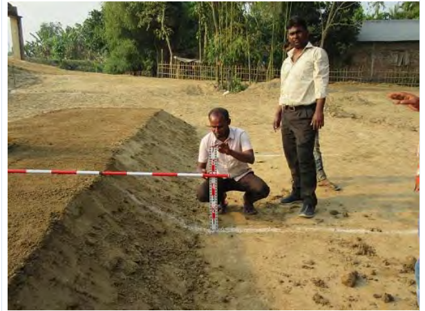
PhD. Check the spreading thickness of 30cm.
