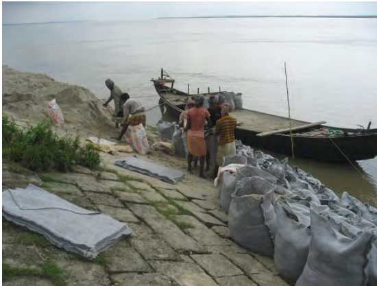
Photo 4.1.1 On-site geo bag sand packing
