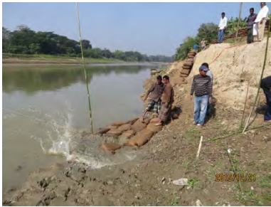
On 21 Dec 2015, dumping S-C GB started from the down stream
