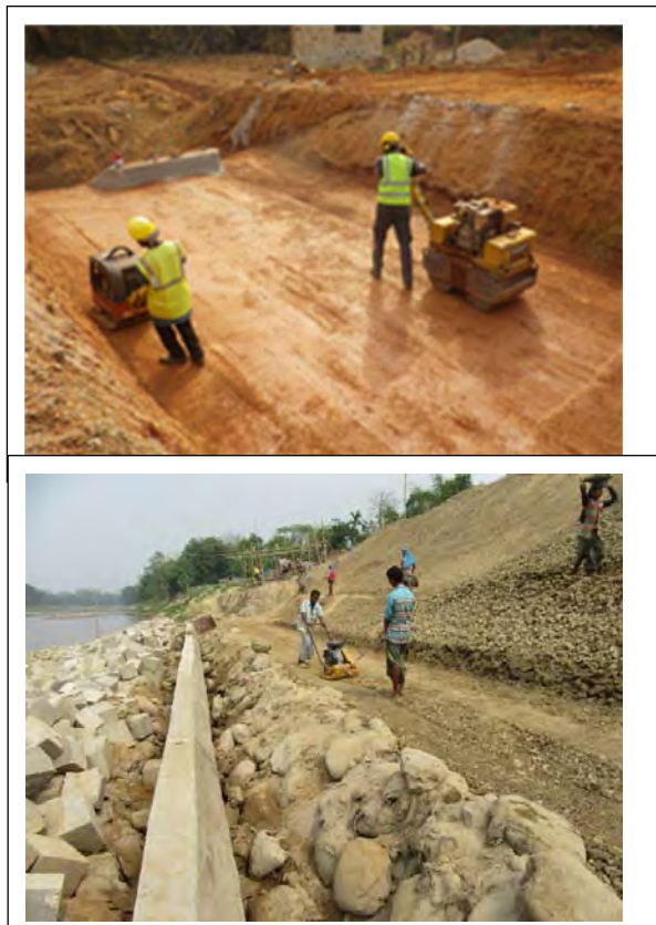
Photo 3.4.3: Compaction using a hand-roller, Plate vibrating compactor & tamper
