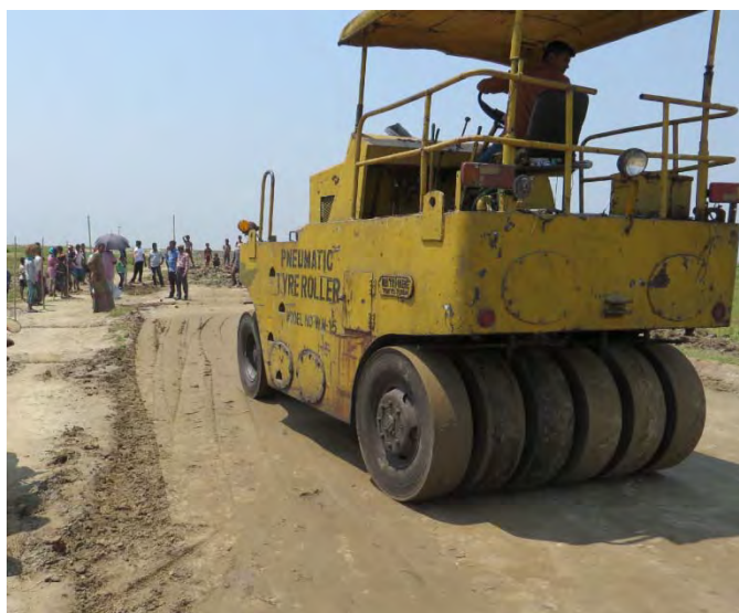
Photo3.4.2 Compaction by tire-roller
