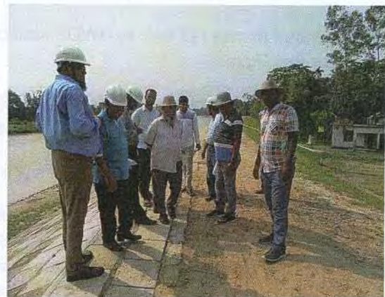
Ph2. Pointing out some sinking part at the embankment crest at around C/S No.16 on Site Inspection
