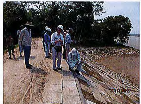
Ph5. Checking construction joint between placing cc-block on cracks and Gap concrete at about C/S # No.16
