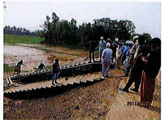
Ph3. Old and new RCC Stair Case on to the Slope near the School.
