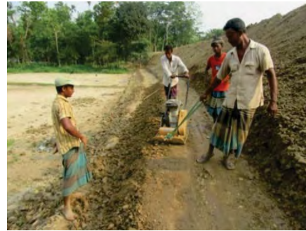
Photo 3.10. Embankment country side slope compacted by plate compactor (on 15 April 2017)
