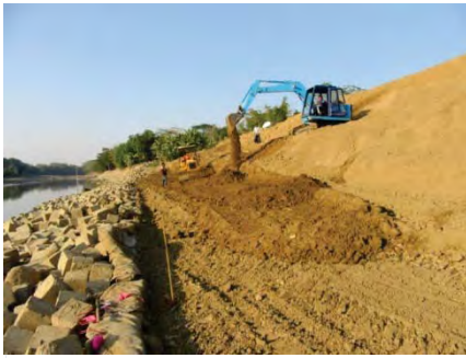
Photo 3.6. Bulldozer and Excavator working/ compacting at slope on 19 Jan 2017
