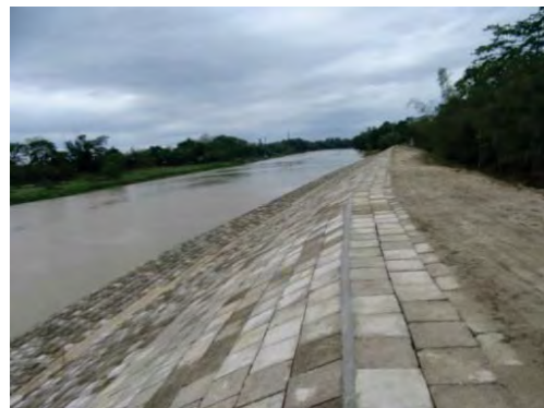
Photo 3.9: Completed Slope Protection from middle toward downstream view on 30 March 2017
