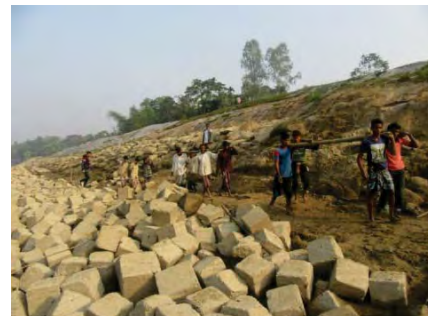
Photo 3.5. At up-stream, salvaging geo-bags WL=5.42m (PWD) on 24 Dec 2016
