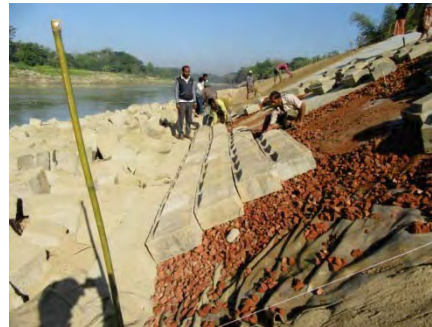
Photo 3.7. Slope protection; sand mat, geo- sheet & CC-block, on 26 January 2017
