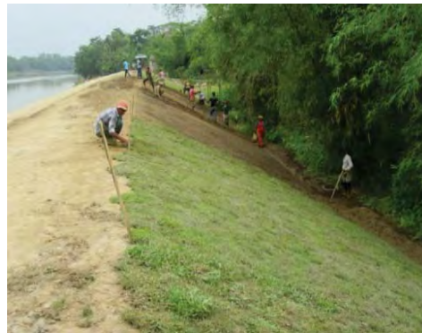
Photo 3.12: Dressing and turfing on country side slope (13 May 2017)
