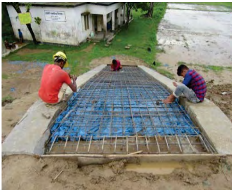
Photo 3.11 Top layer M S reinforcement for StairCase. (on 22 April 2017)
