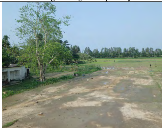
Demobilization work started at stock yard next to the primary school
