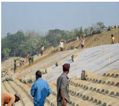
Photo 3.8: Slope protection; sand mat, geo- sheet & CC-block (on 02 Feb 2017)
