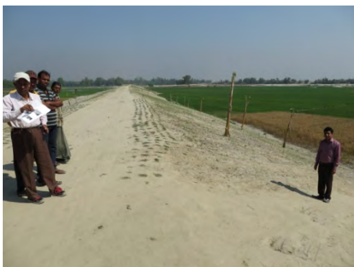
No CC-block protection on slope at retired bank construction in Bogra District
