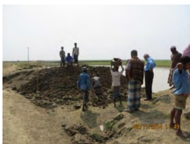
Repair work of submersible embankment in Haor, Netrokona
