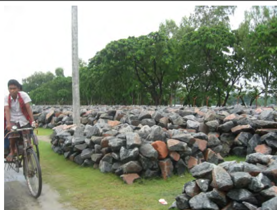
Stockpiled crushed rocks for rehabilitation works of the hard-point at Sirajganj
