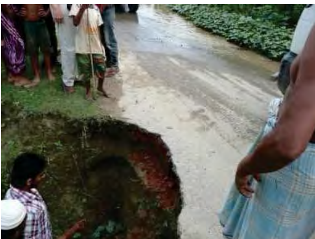
c. failure of river embankment
