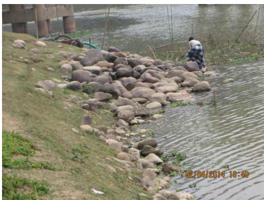
a. Foot protection works with boulders
