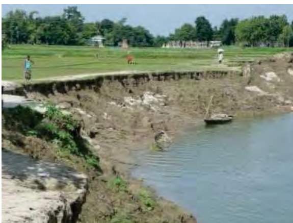
c. Embankment erosion on the city side in the downstream reaches of TPW.
