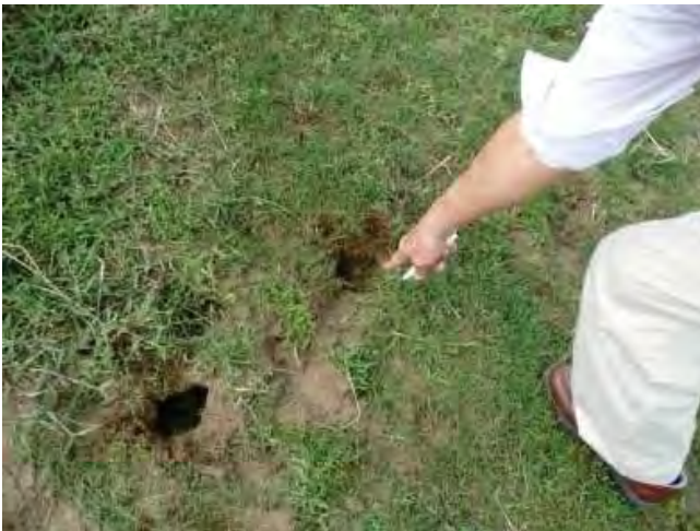
b. rat holes on the river embankment
