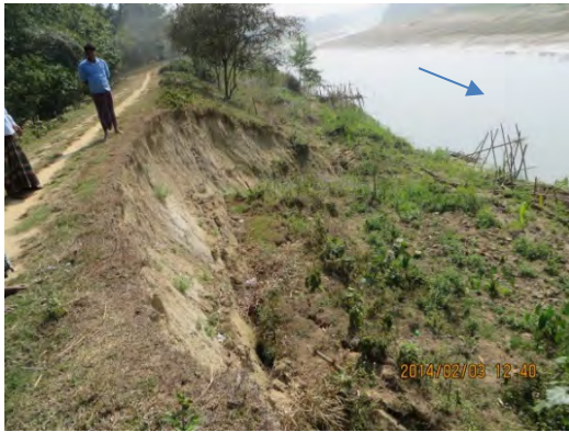
Embank erosion at Moulvibazar; Manu River
