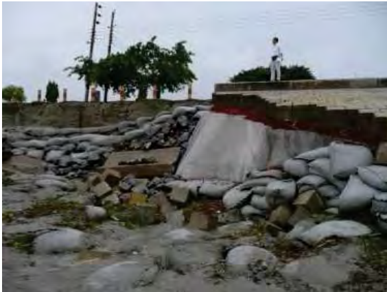
a. River embankment failure site
