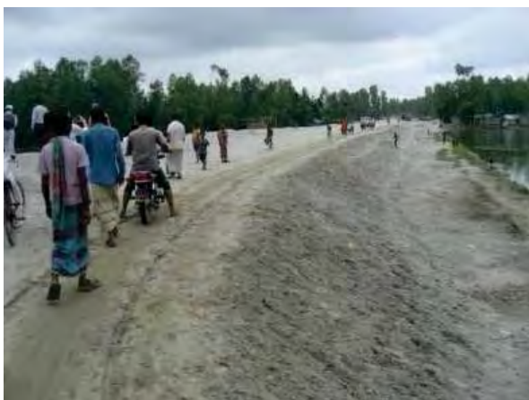
c. New set-back embankment under construction
