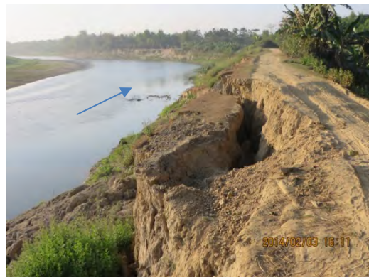
Embank erosion at Moulvibazar; Manu River
