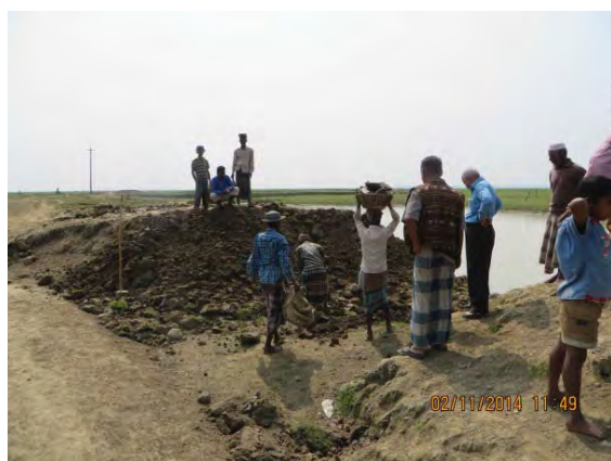
b. Submergible embankment under repairing works
