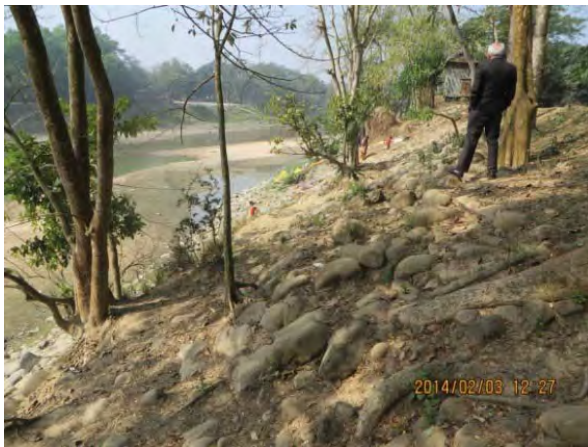
a. Embankment protection with boulders
