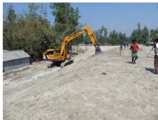
No CC-block protection on slope at retired bank construction in Bogra District
