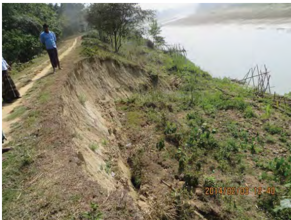
b. Due to the erosion at the embankment toe, the slope slide took place with the scale of 300m long. The embankment crown itself is already very narrow. There exists an elementary school nearby.
