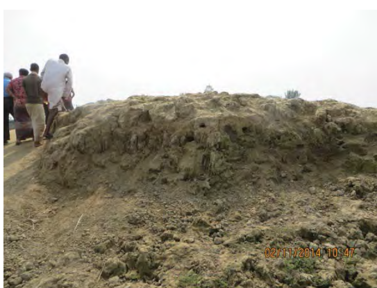
a. Damaged submergible embankment b. Many holes by crabs in the embankment
