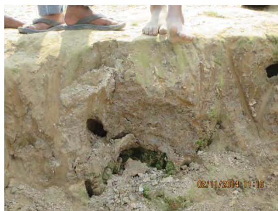
a. Damaged submergible embankment b. Many holes by crabs in the embankment
