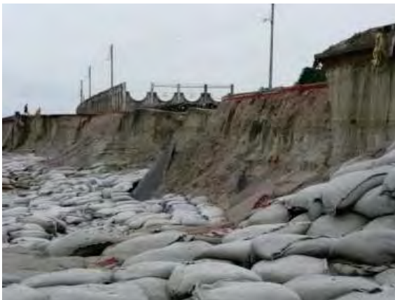
b. many sandbags used for emergency works
