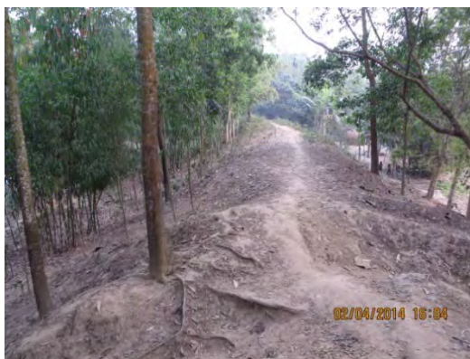
b. Damaged embankment due to the human traffic
