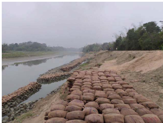
Photograph-4: Pilot Repair Works (as of 23/Jan/2016)
