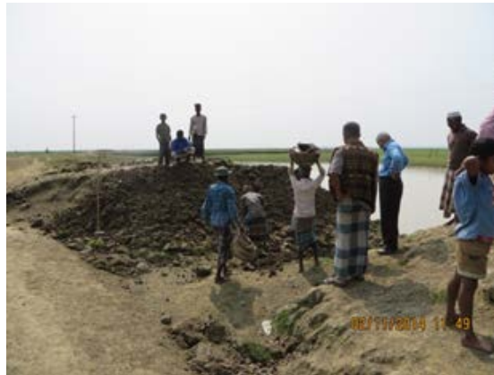
Photograph-2: Reconstruction of Embankment (Netrokona)
