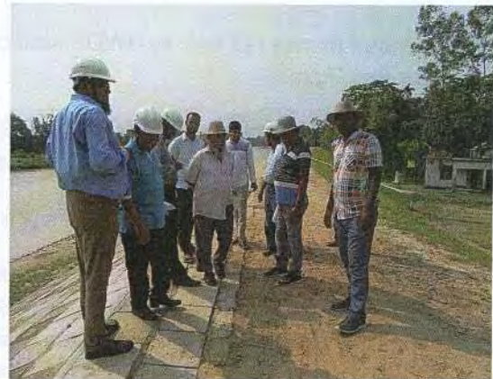
Ph2. Pointing out some sinking part at the embankment crest at around C/S No.16 on Site Inspection
