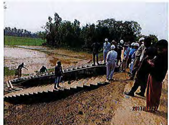
Ph3. Old and new RCC Stair Case on to the Slope near the School.
