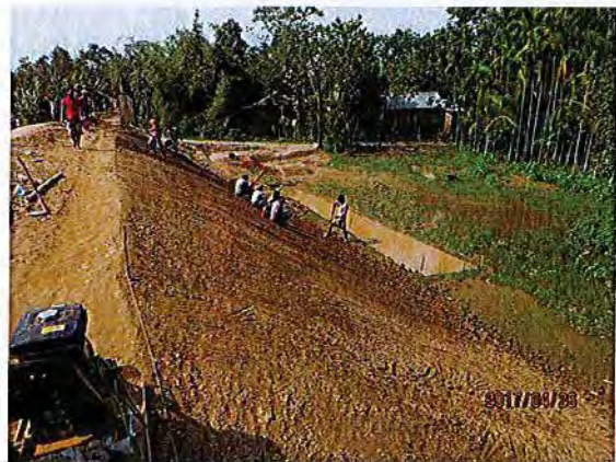
Ph2. Proposed Drainage at Toe of proposed country side slope. Existing swamp small ponds.
