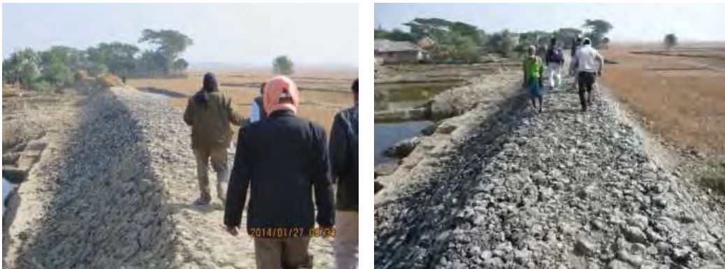
b. Retired embankment under construction by local government
