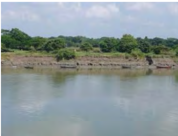
b. Embankment erosion on the other side of the city
