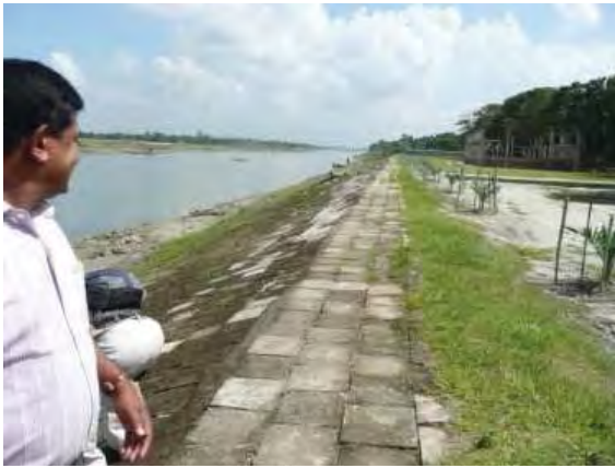
a. Embankment by Town Protection Works
