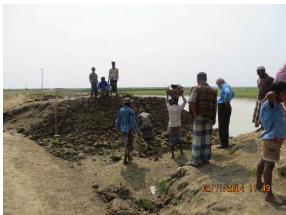
b. Submergible embankment under repairing works
