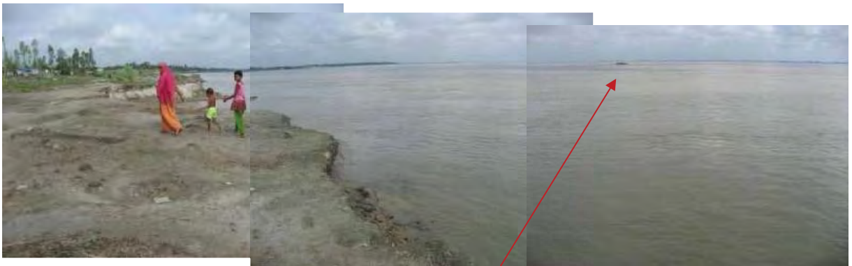
b. the remnant of spur dyke lost in 2004 and 2012 floods
