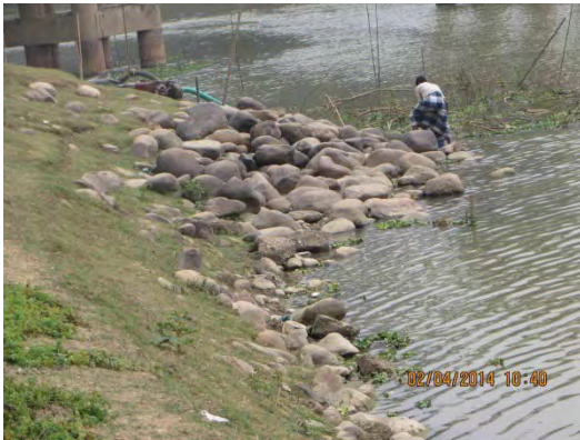
a. Foot protection works with boulders
