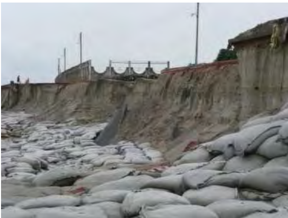
b. many sandbags used for emergency works
