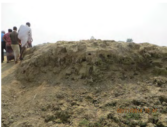
a. Damaged submergible embankment
