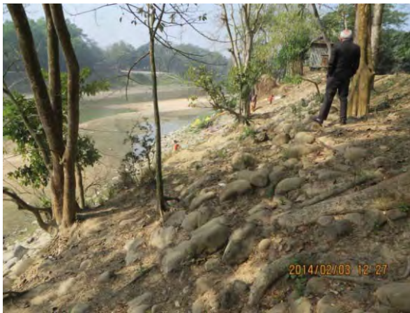
a. Embankment protection with boulders
