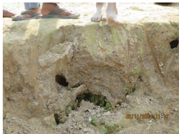
b. Many holes by crabs in the embankment
