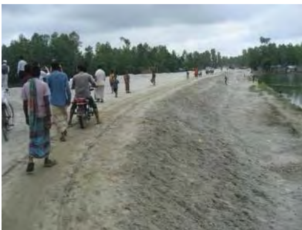
c. New set-back embankment under construction
