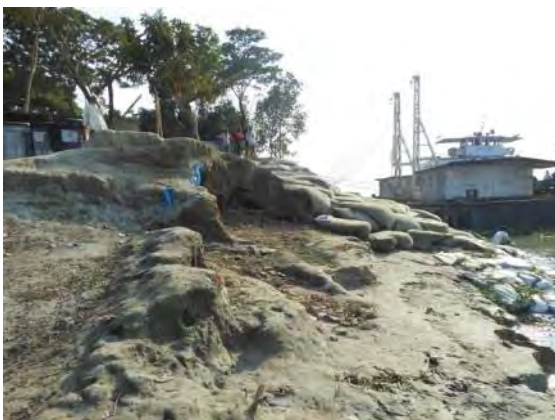
b. Emergent bank protection works (river bank material consists of silt with clay)
