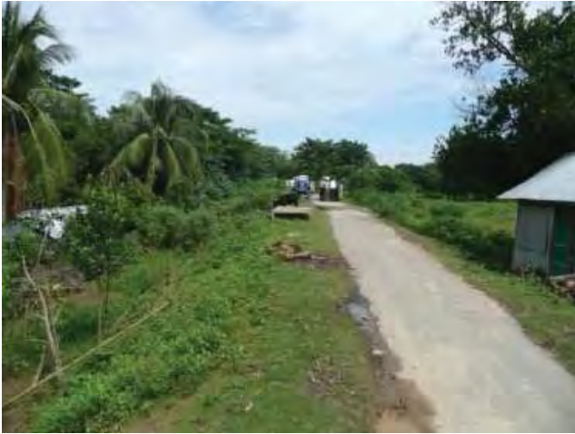
a. general view of river embankment
