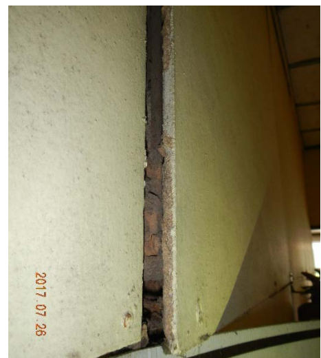
写真：Cement Asbestos Board with Vinyl Paint Finish
