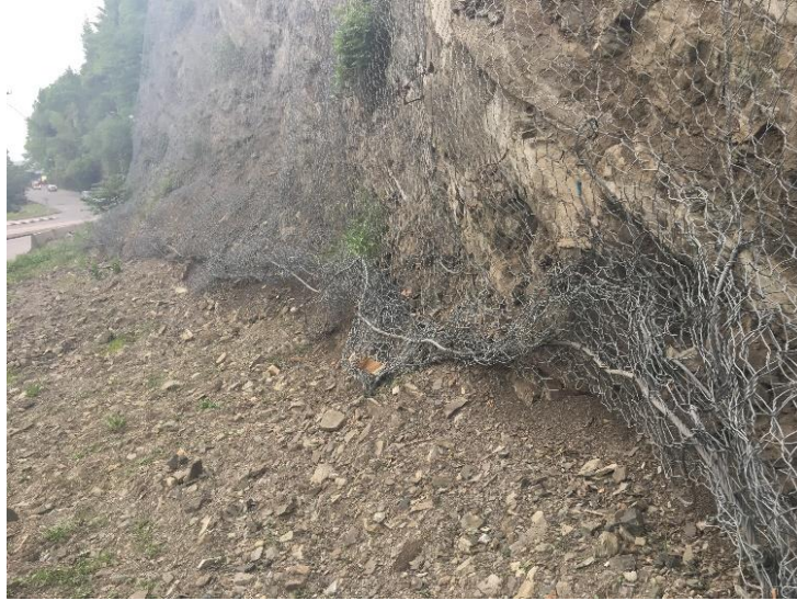
Fig. 4-13 Status of installed measures
