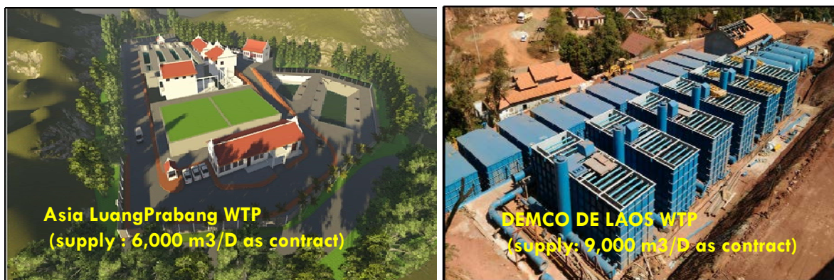
Figure 6-5 Water Treatment Plant using the BOT method
