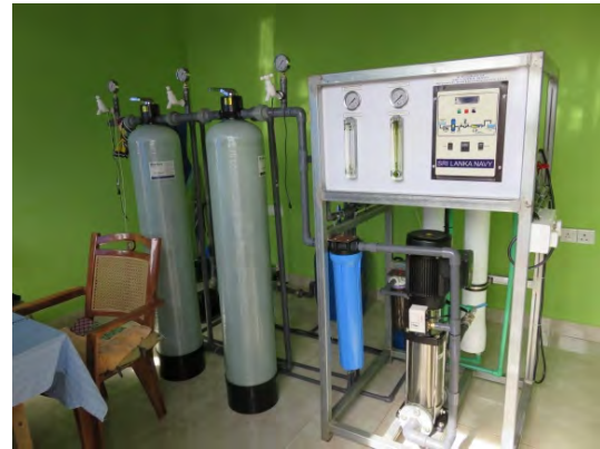
R.O. facility installed by the navy in November 2016. 9 hours operation in a day produces 3,000 liters of water. It is maintained by the navy.
