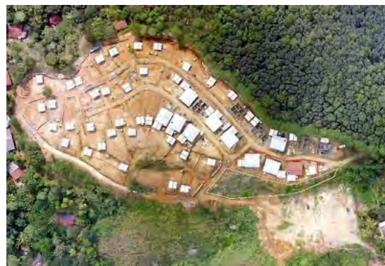
Monitoring of construction using drone
