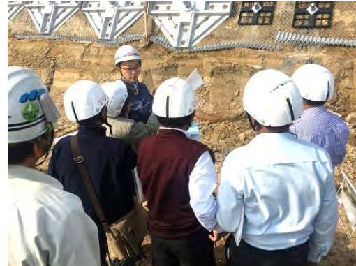
Site visit to slope stabilization site
