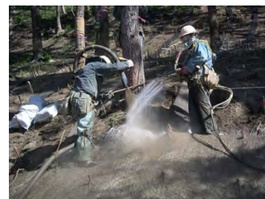
Construction keeping existing trees Source: Nittoc Construction Co., Ltd. HP
