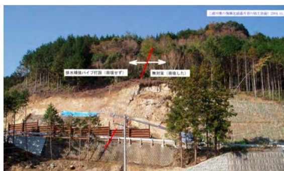
Left: no slope failure in PDR applied slope / Right / slope failure in PDR unapplied slope
