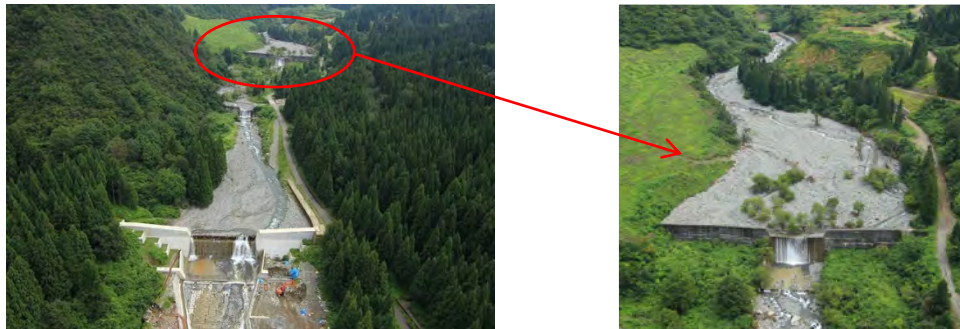
Trapped sediments by Sabo-Dam at Nigata Prefecture, Japan Source: TCLMP
