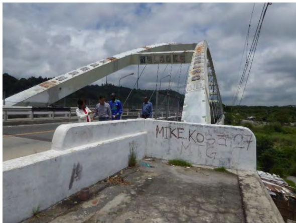
Site visit: Bamban Bridge (Steel Nielsen-Lohse Bridge, Region III)
