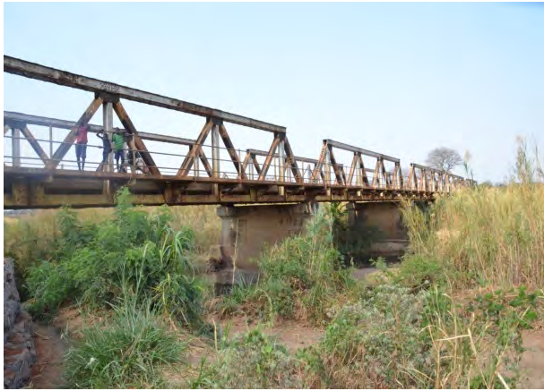
Figure II-27 Corrosion of Steel Truss Bridge
