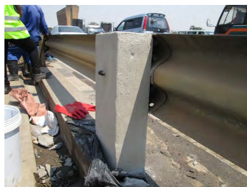
Restoration of guardrail pillars using concrete; application of coating for durability
