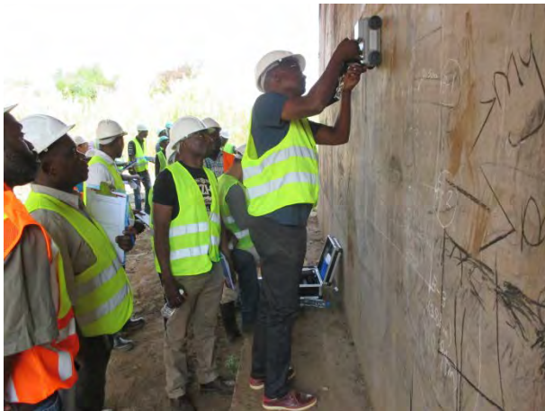
NDT(Rebar Detective Test) Drill
