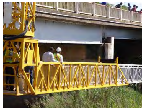
Inspection using the ladder of BIV
