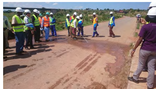
Participant experienced demonstration of expansion joint cleaning by high-pressed water
