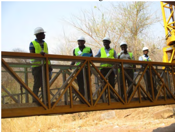
Inspection by BIV
