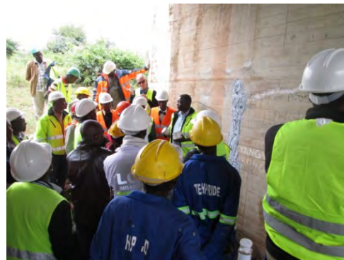
Site demonstration of crack injection on abutment wall in T04-03 bridge
