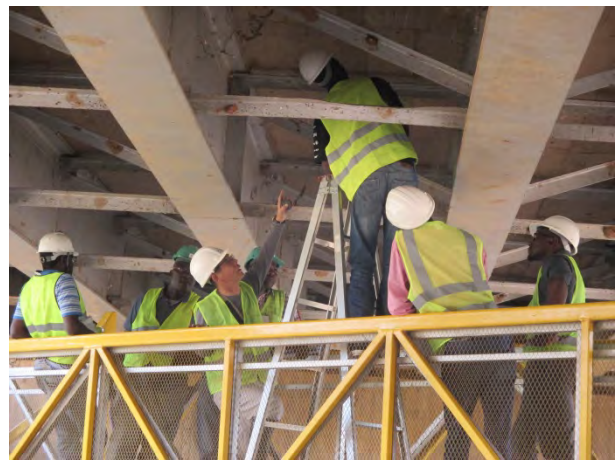
NDT(Rebound Hammer) Drill
