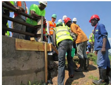
Concrete patching work using polymer cement mortar produced by chemical maker
