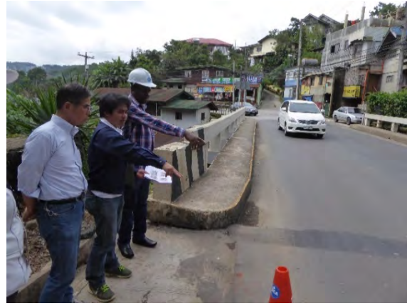
Site visit: Loakan Bridge (Region CAR)
