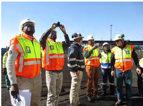
At the Silo Repair Project Site
