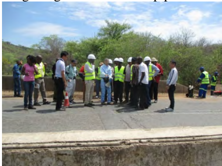
Technical instruction on routine inspection; settlement of abutment damages expansion joint.
