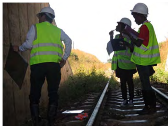
Inspection Activities in Central Province (Trunk Road 2 Br No.304)
