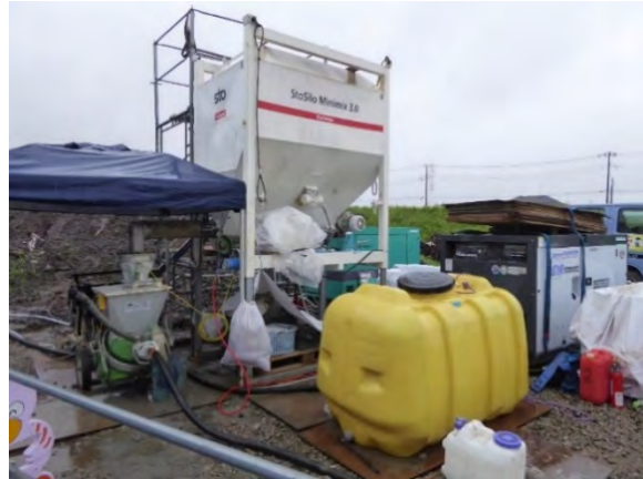
Construction Equipment of Spray Method (Tamamo Bridge Viaduct)
