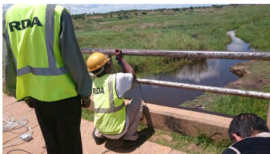
Surface preparation using electric grinder for repainting guardrail
