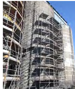
On-going Silo Repair Project Site
