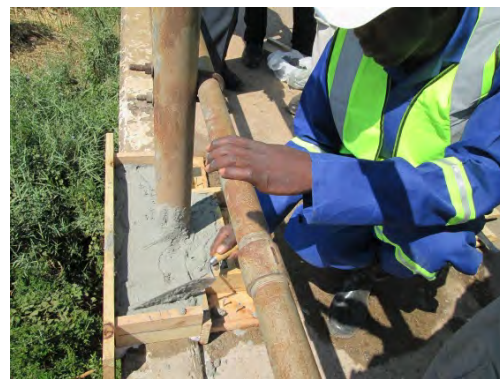
Concrete patching with polymer cement application. Pour and finish by trowel.
