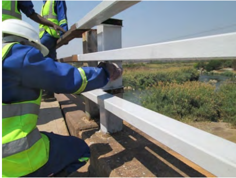
Applying epoxy primer; after drying, finish with polyurethane topcoat.
