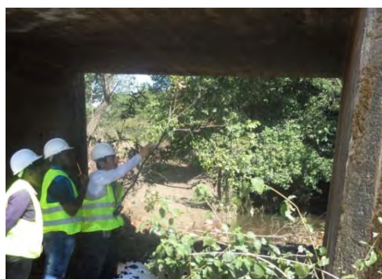
Inspection Activities in Eastern Province (Trunk Road 4 Br No.18)
