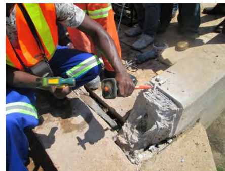
Preparatory work for concrete patching; anticorrosive agent already applied to rebars
