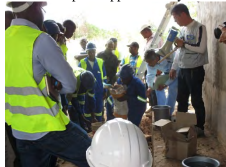
Technical instruction on concrete patching; mixing polymer cement with water
