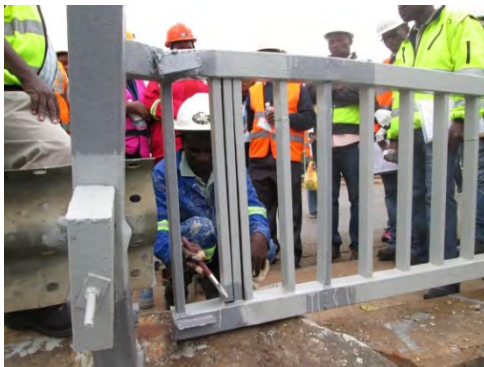
Site demonstration of re-painting on guardrail in T04-02 bridge
