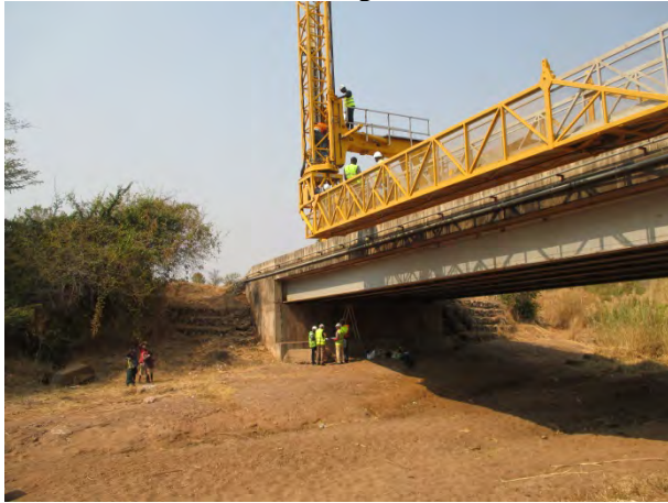
Inspection by BIV
