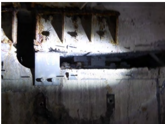
Replacement of Bearing (Existing) (Metropolitan Expressway No.4 Route)
