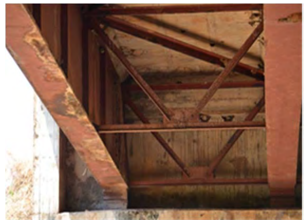
Corrosion due to water leakage
