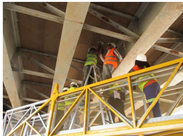
NDT(Rebound Hammer) Drill
