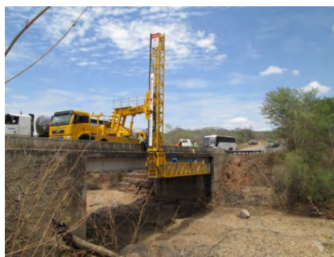
Cleaning girders using BIV at Monthly Site Visit Meeting
