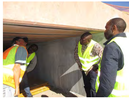
Bridge Repair Project Site in Upington
