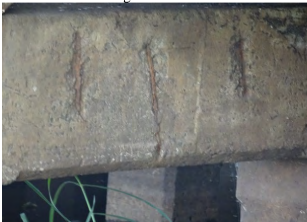
Figure II-28 Damage on Concrete Girder
