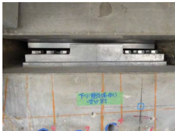
Replacement of Bearing (New) (Metropolitan Expressway No.4 Route)
