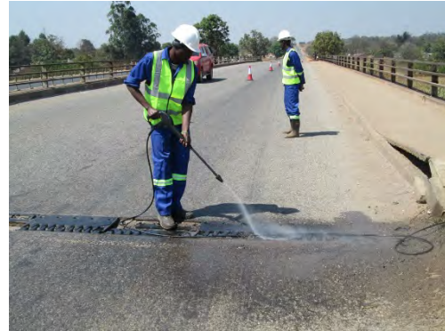
Cleaning expansion joint with high-pressed water cleaner.
