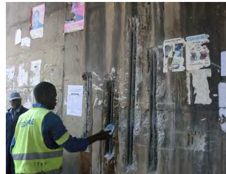
Works of concrete patching
