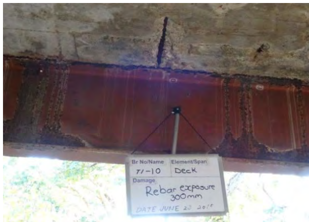
Corrosion due to water leakage
