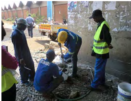
Works of concrete patching
