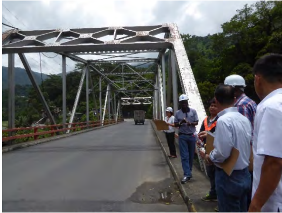
Site visit: Camp 4 Bridge (Region CAR)
