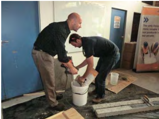
Repair Demonstration of Patching in BASF (Mixing of Material)
