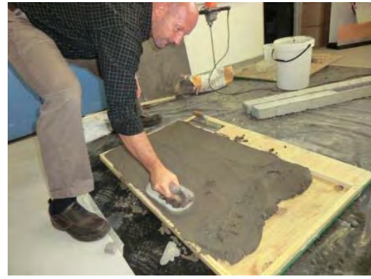
Repair Demonstration of Patching in BASF (Trowel finishing)
