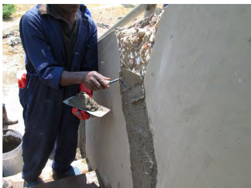
Concrete patching, applying polymer cement mortar using metal trowel
