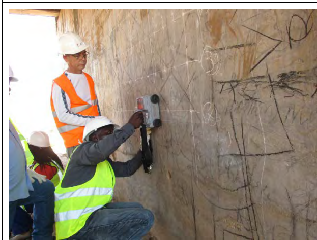
NDT(鉄筋探査計)実習
