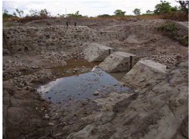
Downstream view of the weir: Main part of stone masonry weir was completed. MWS 6-1 Buyamntanishi, November 11, 2014.
