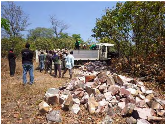
Ferrying stones : Stones were ferried from quarry site to the construction site by a truck. MPR 14-1 Mpela. September 11, 2014
