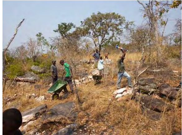
Breaking stones: Stones were gathered near the site breaking rocks. MPR 14-1 Mpela. August 29, 2014
