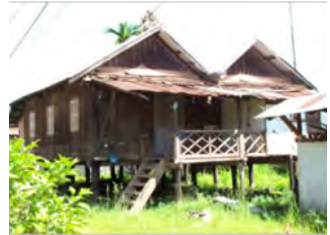
Photo: Lao traditional building
