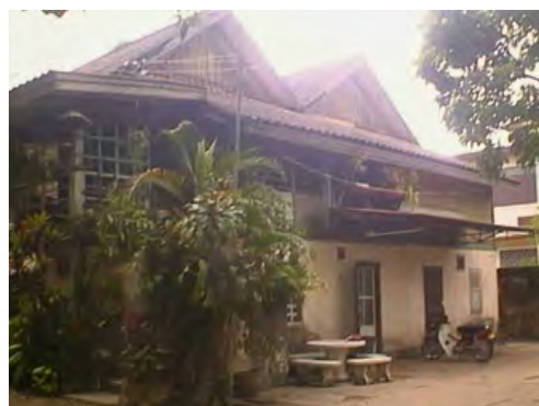
Photo2: Lao Payouk Buildings (Source: Vientiane, portrait d'une ville en mutation: Chayphet Sayarath)
