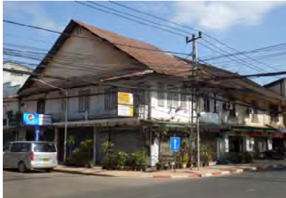
Row House with Lao Conventional Construction Method
