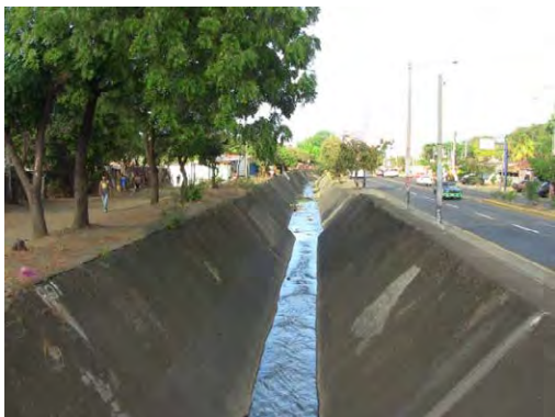
Along the right bank of the cauce is one main highway: the Pista Juan Pablo II.
