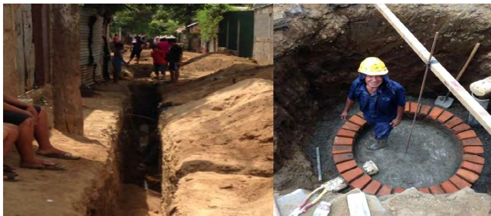
Figure 5.3.5 Condominial Sewer System, Manhole Construction at Villa Reconciliacion Sur
