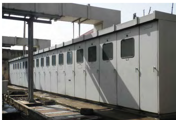
Figure 4-19 15kV Switchgear Panels
