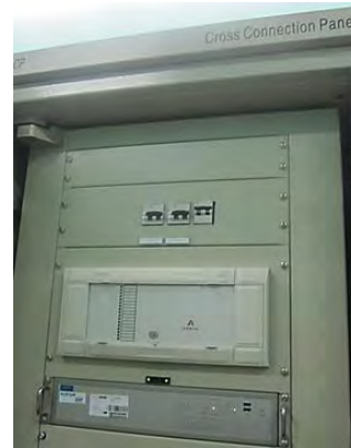
Figure 4-13 Existing RTU (Micom C264)
