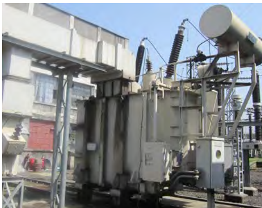
Figure 4-1 Power Transformer
