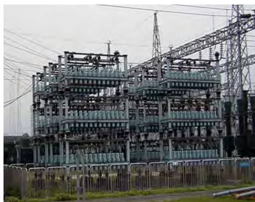
Figure 3-18 Can Type Capacitor
