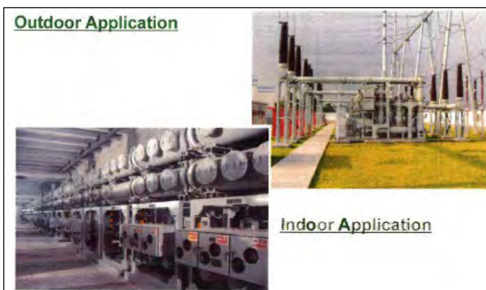
Figure 3-19 An Example of Outdoor and Indoor Type GIS
