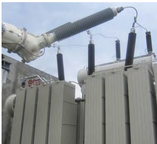
Figure 4-6 ADE S/S Power Transformer and GIS
