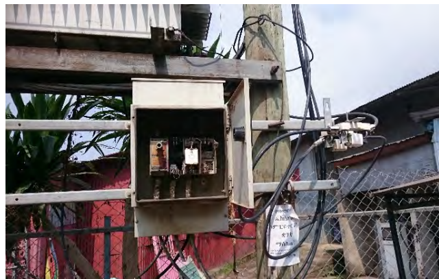
Status of protection fuse for transformer secondary side
