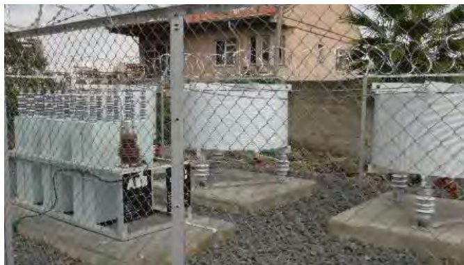
Figure 4-38 15kV Capacitor in Addis East Substation
