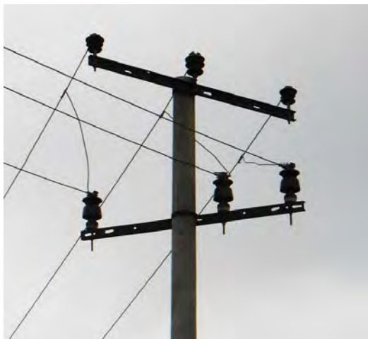
Figure 4-40 Usage Status of Pin Post Insulator (lower row)
