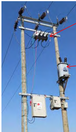
Control source Transformer 33/0.2kV
