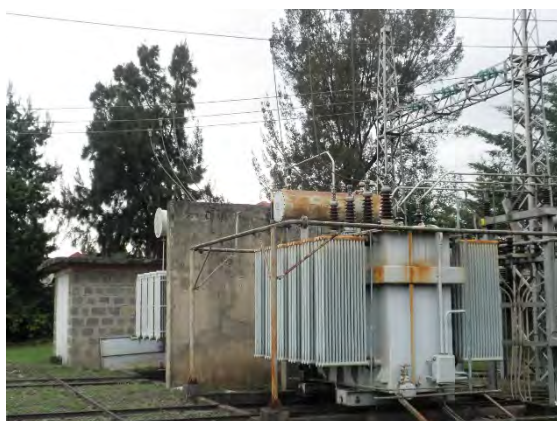
Figure 4-24 Transformer of ADE (6MVA)
