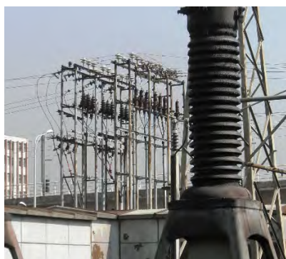
Figure 4-22 Conventional Outgoing Feeder Equipment
