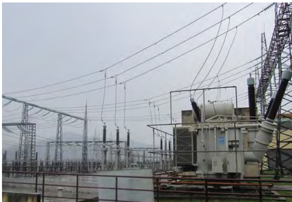
Figure 4-10 Power Transformer 230/132kV
