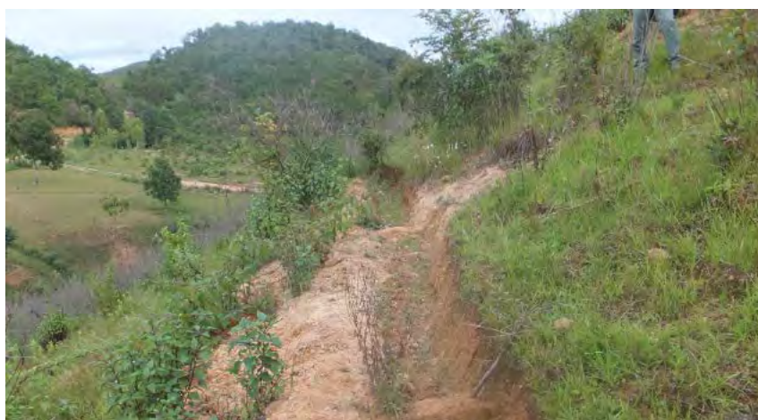
Photo II -22 Trench along contour
