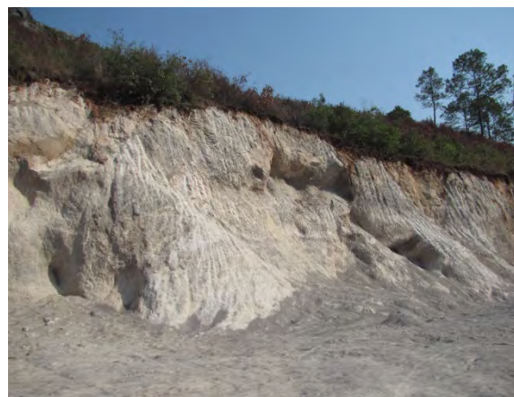
Photo II -13 Surface soil was eroded and foundation soil is exposed.
