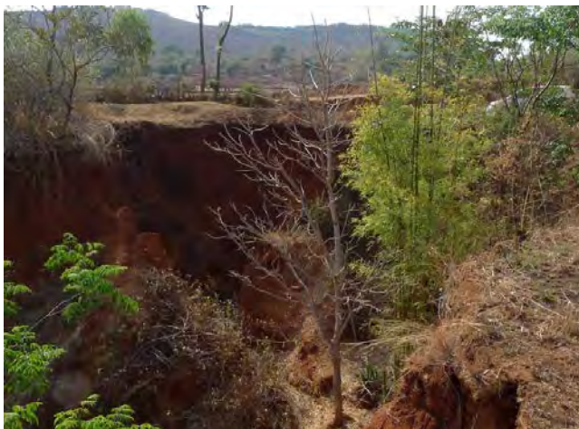
Photo II -10 Gully developed at road side
