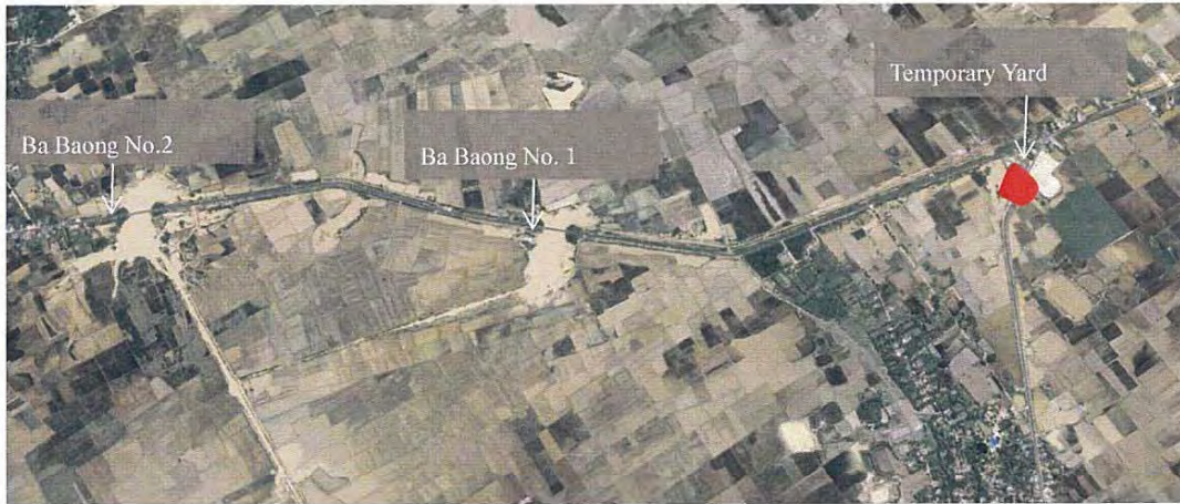
Figure 1-1 Temporary Yard on NR11
