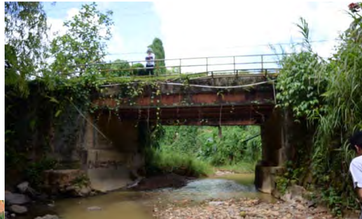
View from downstream
