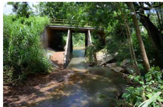
Side View from upstream
