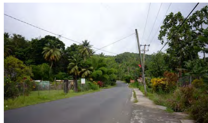
View from the west side AADT 4,800Vehicles/day
