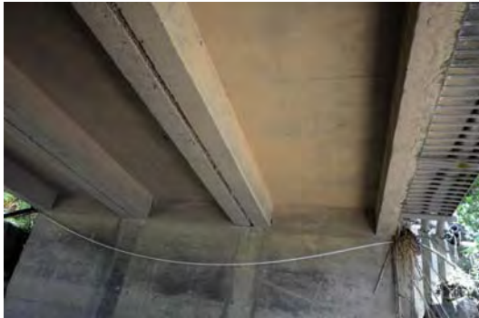
Undersurface of the superstructure
