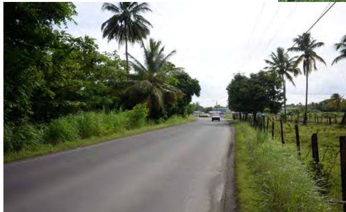
West View from the bridge AADT 8,700 Vehicles/day
