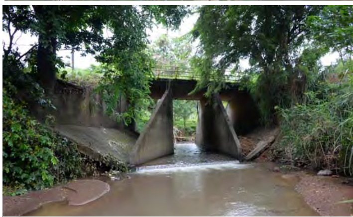
View from downstream
