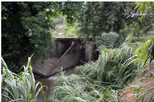
Side View from downstream
