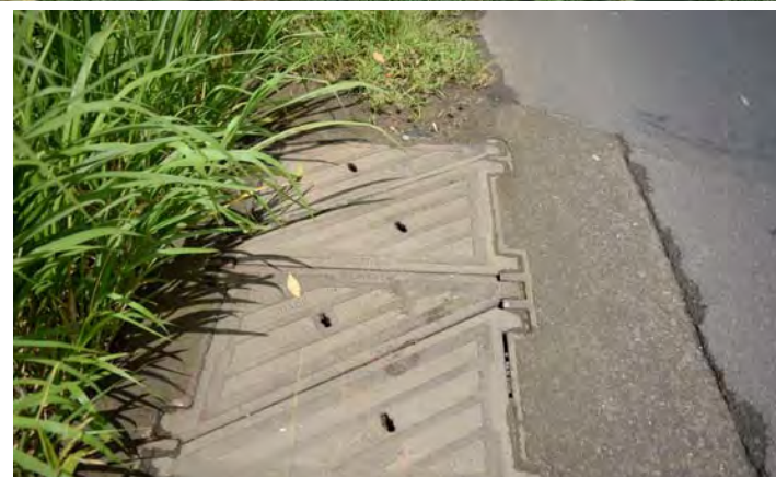
Handhole near the bridge
