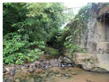
Photo: Confluence with a tributary at d/s of Raviine Poisson Bridge
