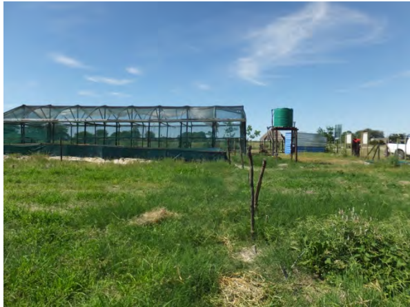
March 2016, site visit. Roof sheets for rain water harvesting
