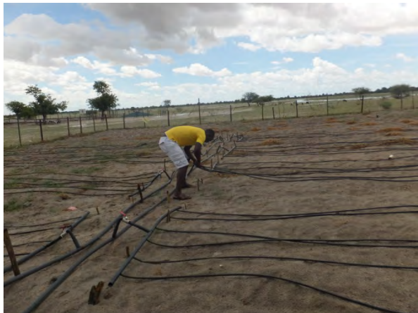
February 2017, installation of drip irrigation
