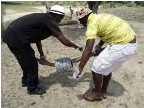
Phase-2. Distribution of fencing materials
