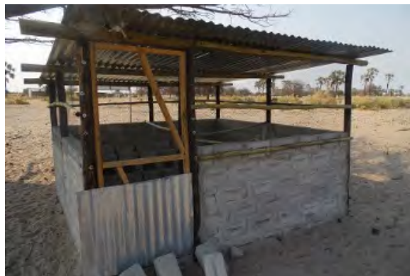
Phase-2. Constructed poultry house
