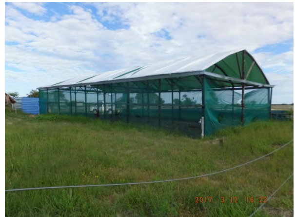
March 2017, under renewal of roof sheets
