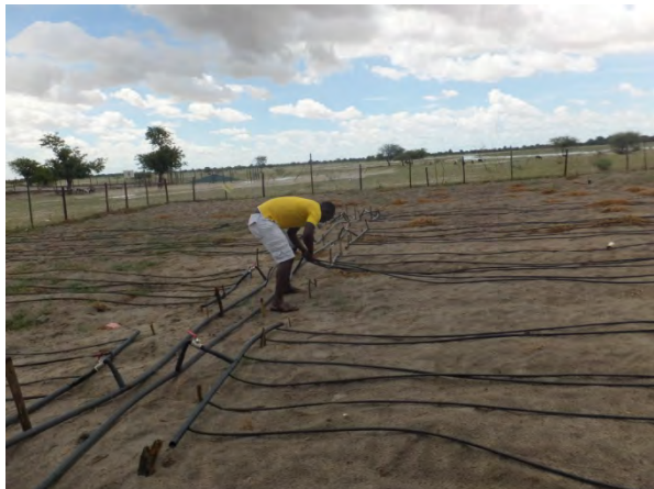
February 2017, installation of drip irrigation
