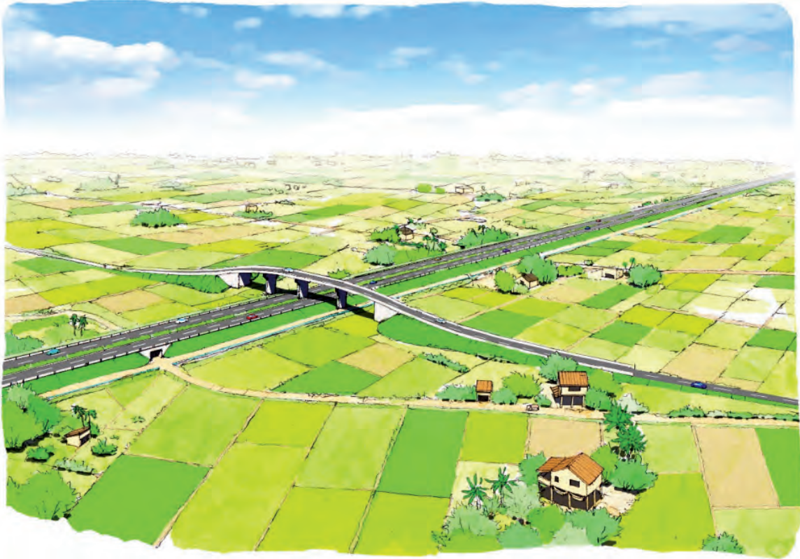
Bird's Eye View of Embankment Section with Over-Pass Bridge, Under Pass Culvert and Frontage Road
