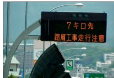
Figure 6-23 Example of Variable Message Board
