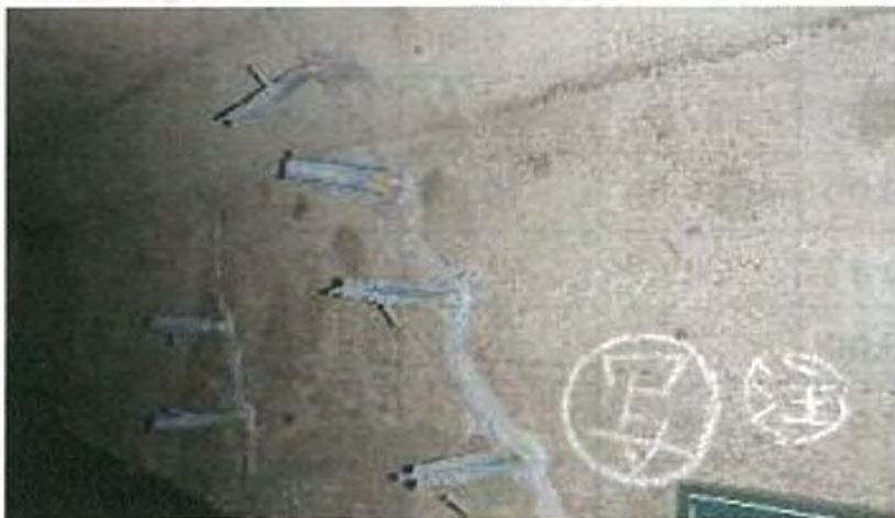
Crack Injection (Side of Beam)
