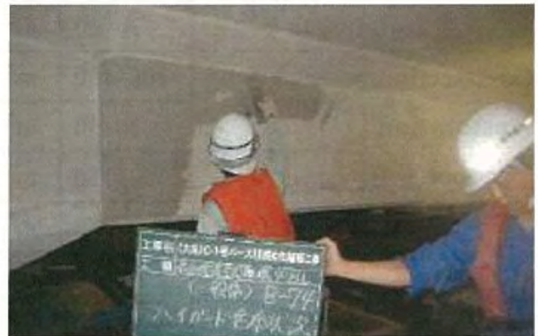
Surface Coating (Side of Beam)
