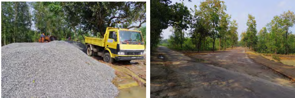
Left : Material Stock at Construction Site of Upazila road in Sripuur
