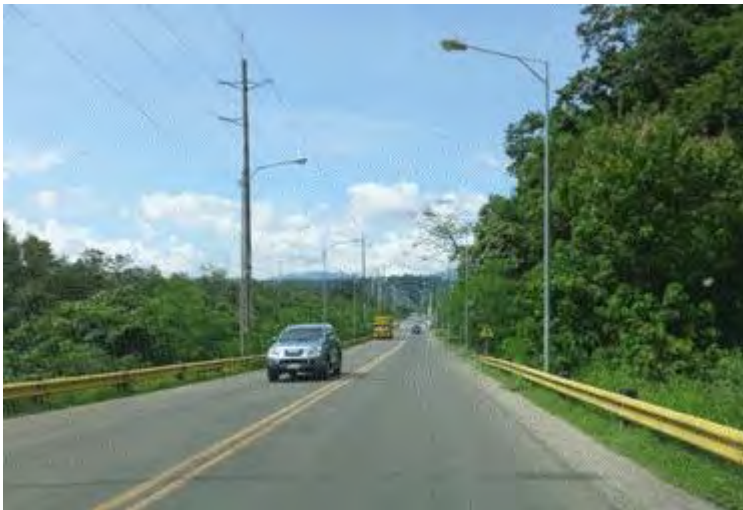
Access road between the Subic Port and SCTEX
