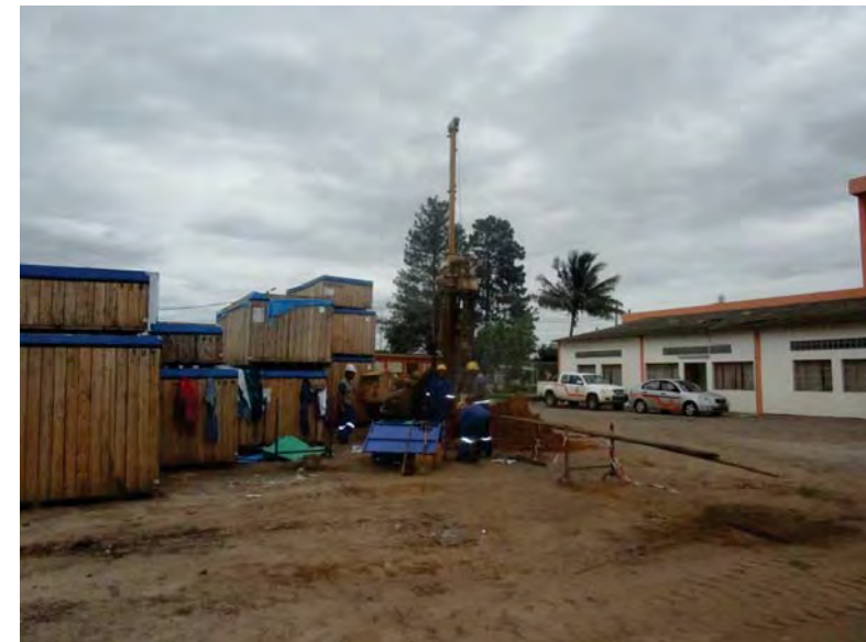
Figure 2 - Drilling rig in borehole 1
