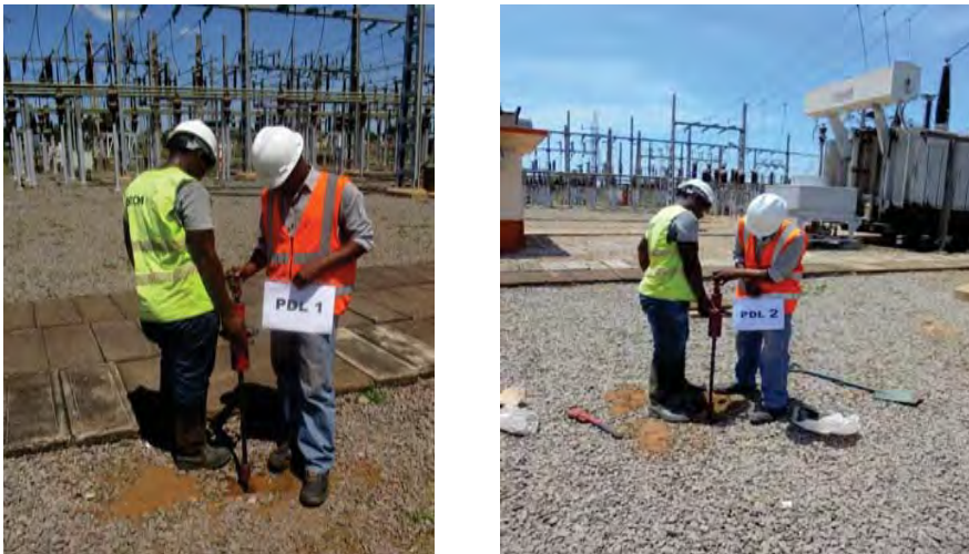
Figure 5 – Illustration of DPL-01 and DPL-02 works at the site
