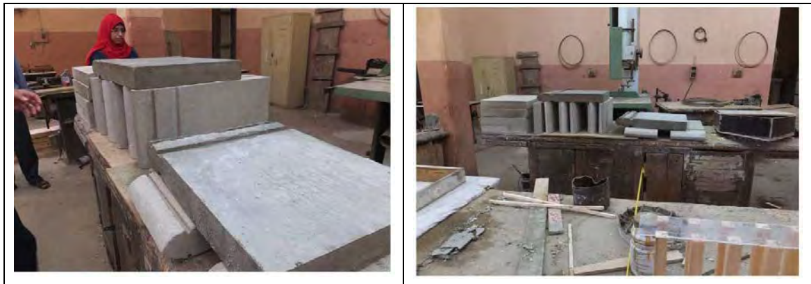
Figure 3-2.7 Scenes of constructing of existing regulators (large scale regulator pier)
