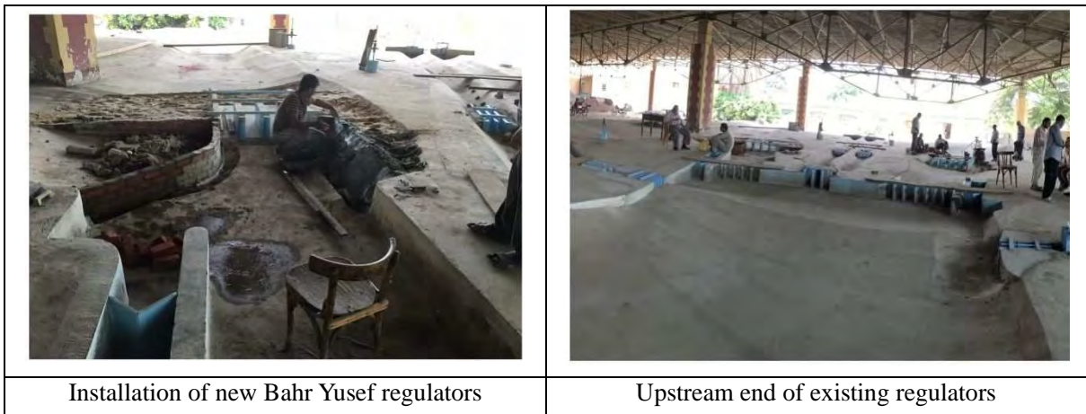
Figure 3-2.17 Installation of new regulators at test site
