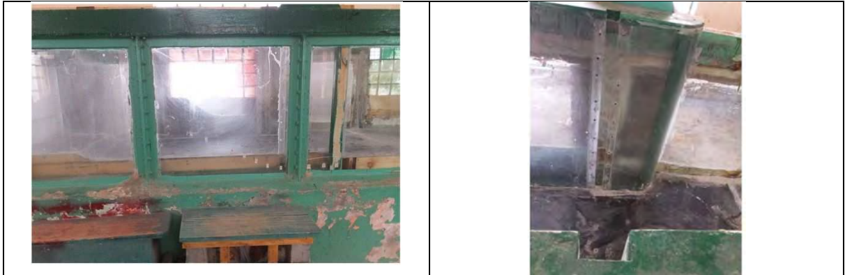
Figure 3-3.9 Installation of regulator piers
