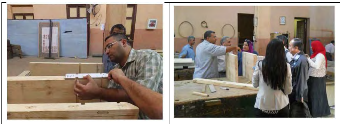
Figure 3-2.6 Scenes of constructing of existing regulators (small scale regulator pier)
