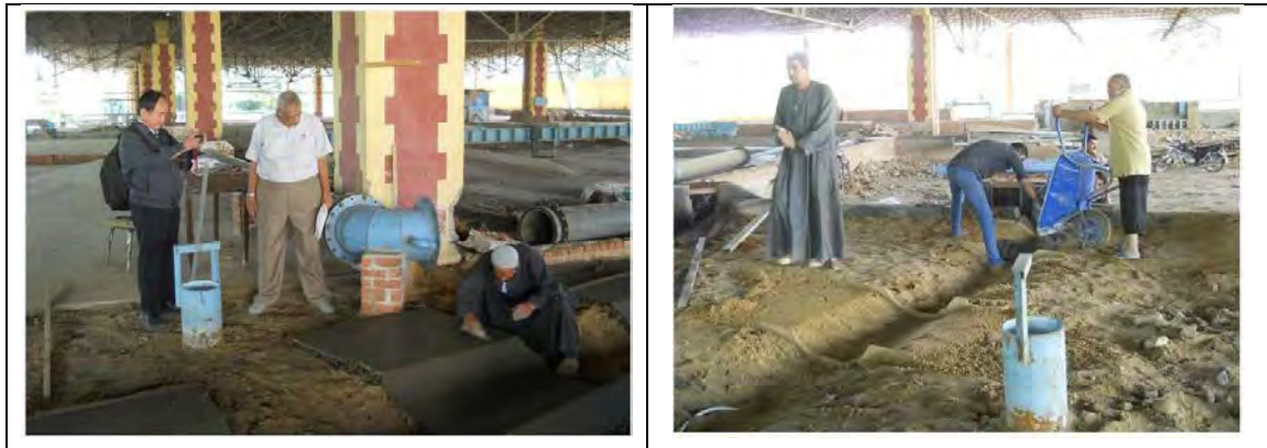
Figure 3-2.8 Scenes of constructing existing canals (using mortar)
