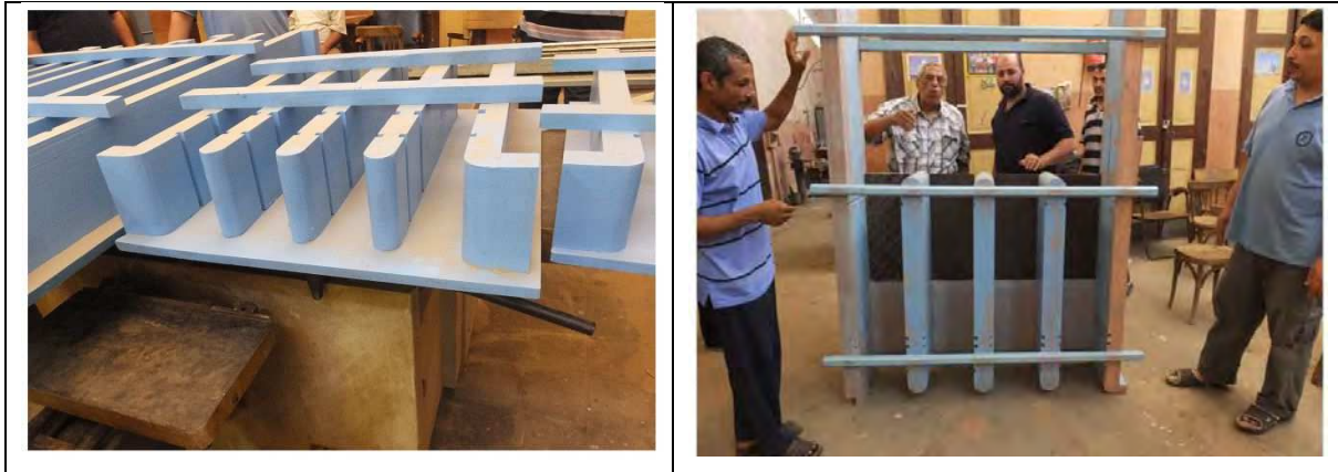
Figure 3-2.16 Scenes of construction of new regulators (large scale regulators)
