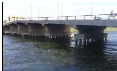
Figure 1-1.6 Upstream view of the existing bridge (No. B18)
