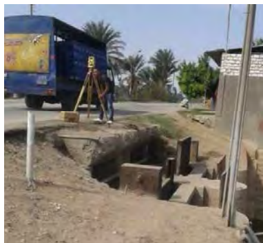
Figure 1-1.7 Photograph of water intake facility
