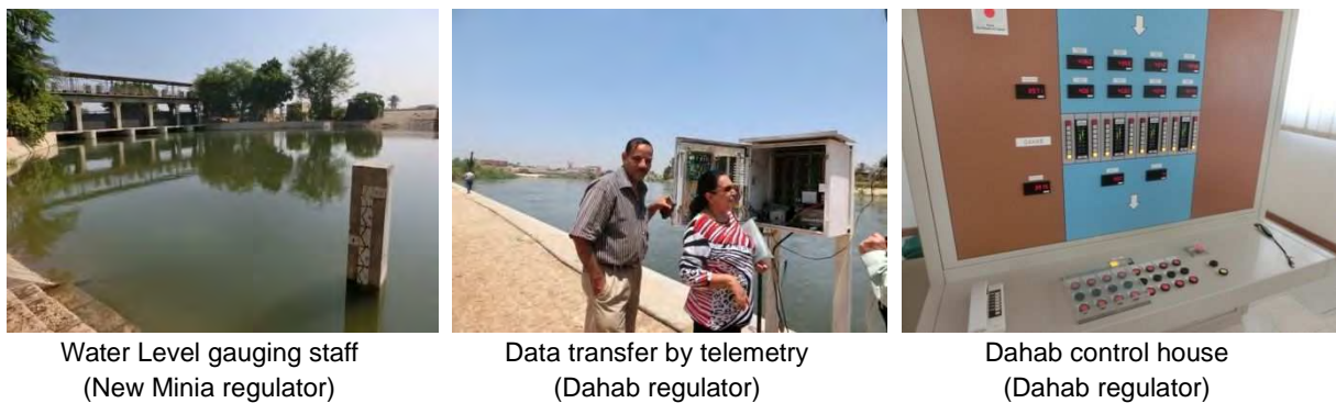
Figure 2-9.1 Existing water level monitoring system (left: a station at the Water Distribution, center: a station of the CDT, right: IIS)
