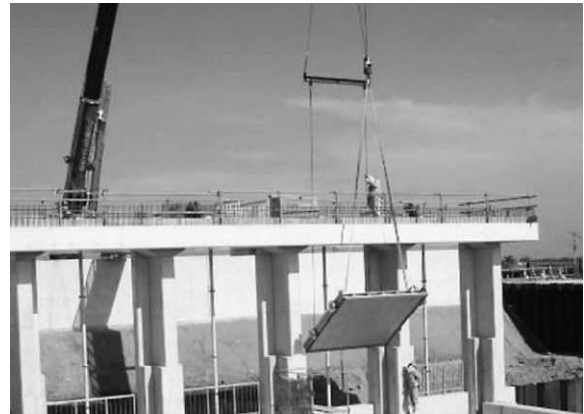
Figure 18-3.1 Hanging method of gate (Small regulators)
