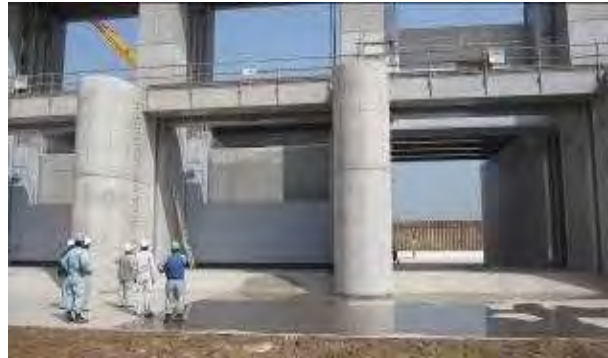
Photo6 : Near view of Double leaf gates (Dahab Regulator)
