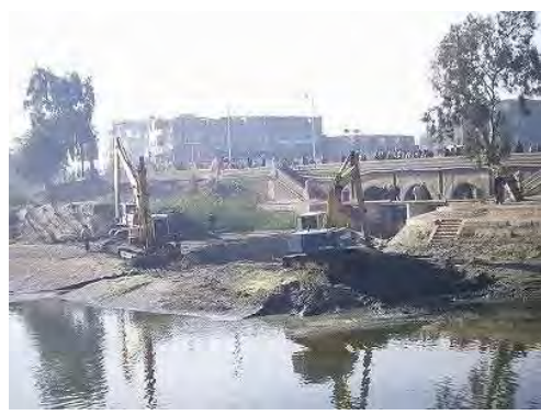
Photo4 : Dredging (upstream of DGRs)
