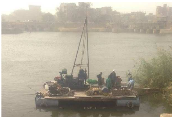
Photo11 : On-water boring on NDGRs axis
