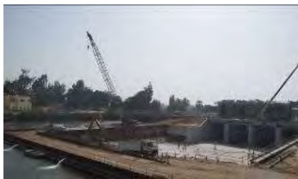
Photo8 : Steel double sheet pile method (Dahab Regulator)
