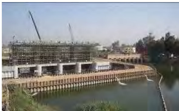
Photo7 : Steel double sheet pile method (Dahab Regulator)
