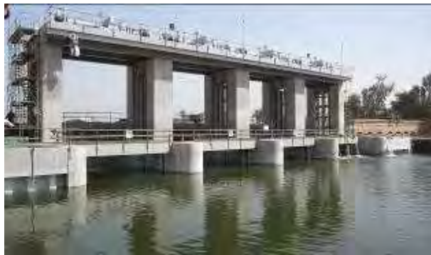
Photo5 : Distant view of Double leaf gates (Dahab Regulator)
