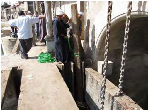
Photo3 : Current Gate Operation (with a log to push the gate)
