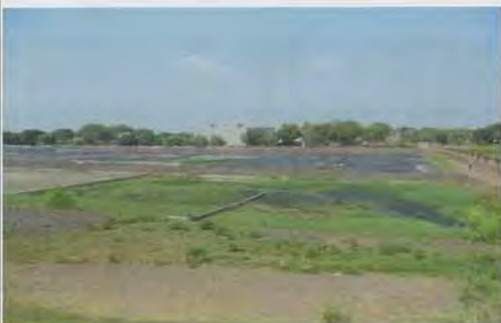
Note) 30-Sep-2015 Varanasi DinapurSTP-5 Drying Bed
