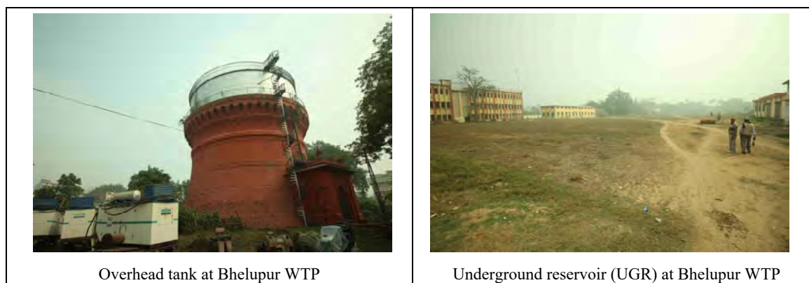
Figure 3.2.5 Water storage reservoirs in Varanasi
