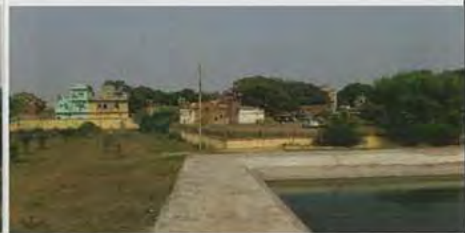
Note) 4-Dec-2015 VindhyachalSTP-4 Aerobic Pond and STP Boundary (Short of walls is STP area.)
