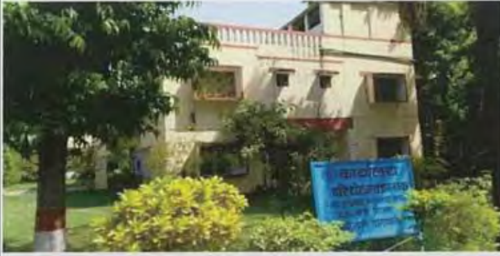
Note) 30-Sep-2015 Varanasi BhagwanpurSTP-1 Administration Building
