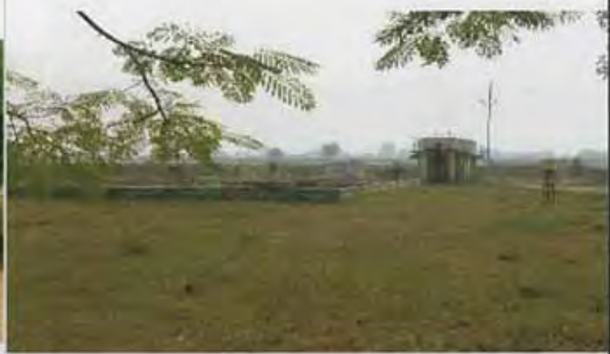
Note) 4-Dec-2015 VindhyachalSTP-2 Inlet Chamber and Sludge Bed
