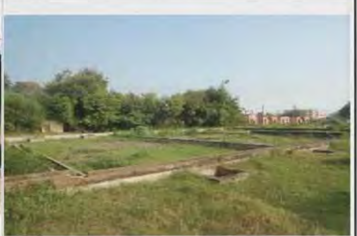
Note) 30-Sep-2015 Varanasi BhagwanpurSTP-6 Drying Bed
