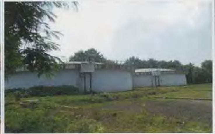
Note) 30-Sep-2015 Varanasi DinapurSTP-4 Digestion Tank
