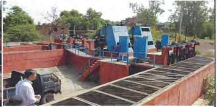
Note) 30-Sep-2015 Varanasi KoniaMPS-4 Screen Chamber
