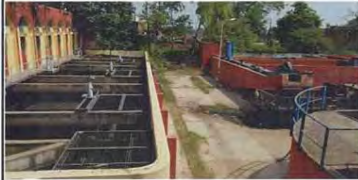
Note) 30-Sep-2015 Varanasi KoniaMPS-3 Distribution Chamber
