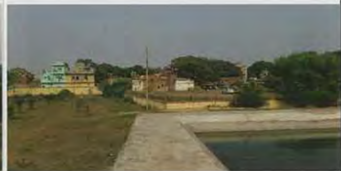
Note) 4-Dec-2015 VindhyachalSTP-4 Aerobic Pond and STP Boundary (Short of walls is STP area.)
