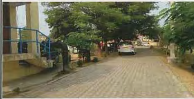
Note) 4-Dec-2015 VindhyachalSTP-1 Entrance Road
