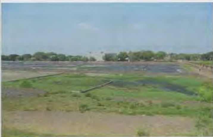
Note) 30-Sep-2015 Varanasi DinapurSTP-5 Drying Bed
