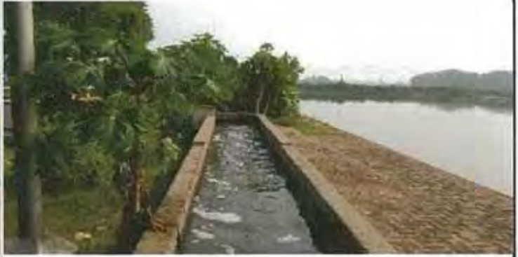
Note) 4-Dec-2015 MirzapurSTP-4 Channel between UASB Reactor and Oxidation Pond
