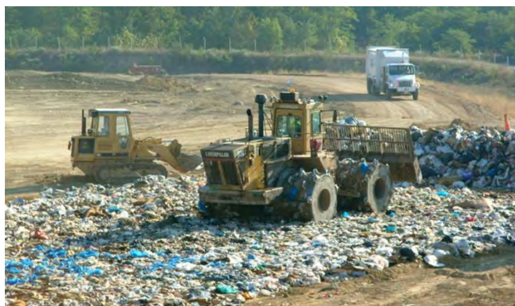
Photo 26 Flat Compaction
