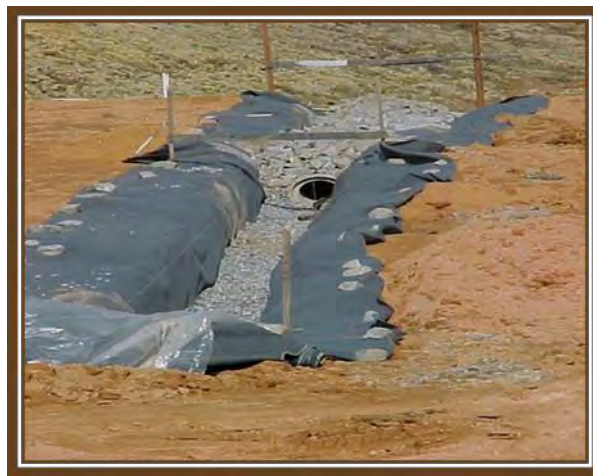
Photo 7 Construction of drains for the collection of leachate
