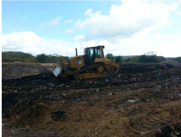
Photo 14 Bulldozer spreading waste in the rehabilitation of the FDS of Azua
