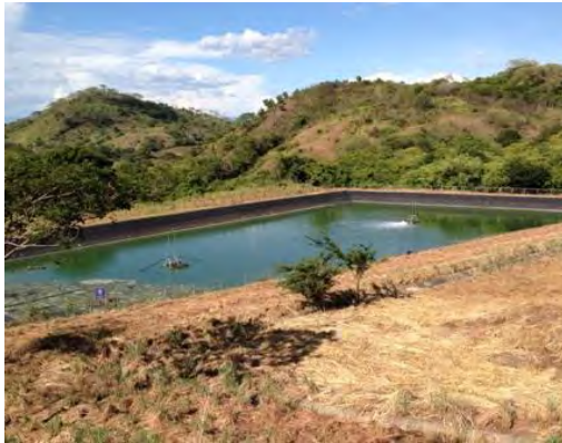
Pond of leachate with waterproofing and sprinklers to reduce bad odors in the Sanitary Landfill of ASINORLU, Santa Rosa de Lima, El Salvador.-
