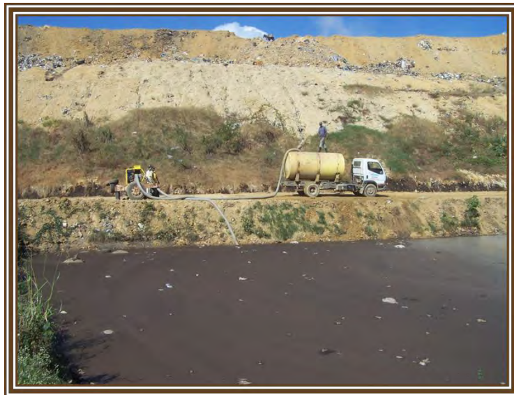
Photo 34 Recirculation of leachate in the waste mass
