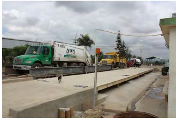
Scale for weighing of waste pick-up trucks at the Duquesa landfill, Santo Domingo, Dominican Republic
