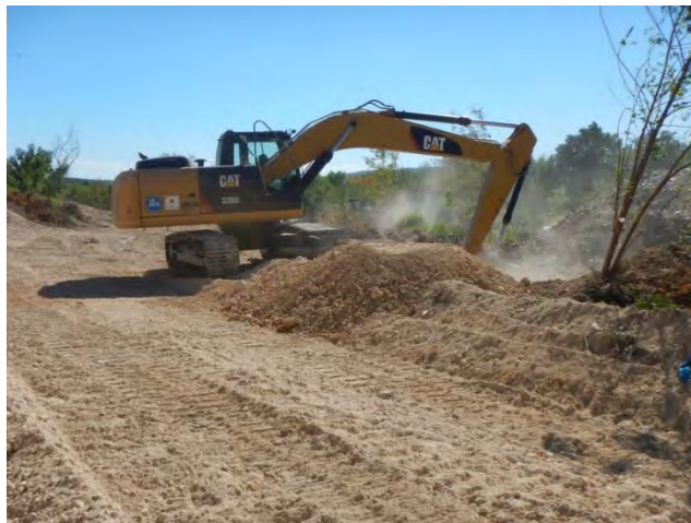
Photo 17 Excavation of cover material at Azua's Dumping Site
