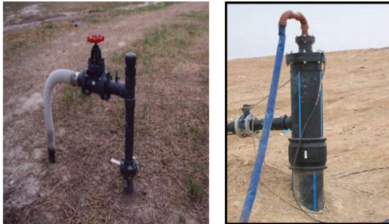
Photo 31 Vertical extraction wells
