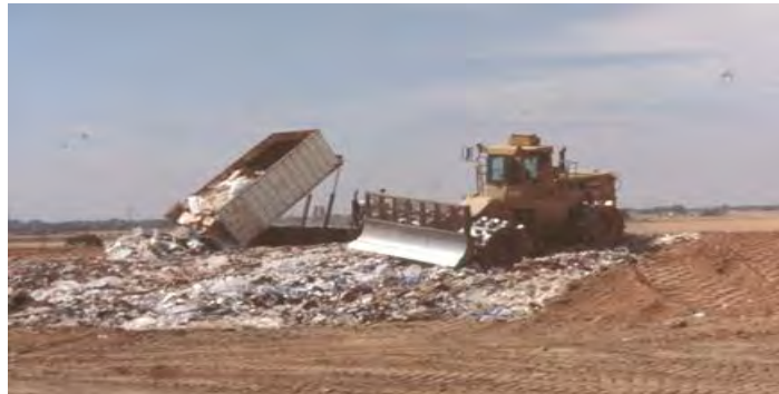
Photo 4 Spreading, compaction and coverage in a landfill
