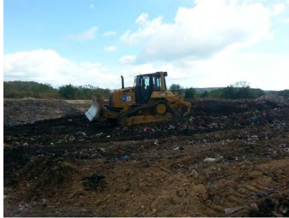
Photo 24 Spreading and compaction of waste with bulldozers in the FDS of Azua
