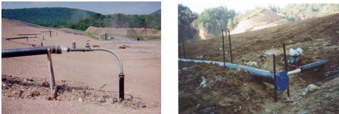
Photo 32 Horizontal extraction wells.
