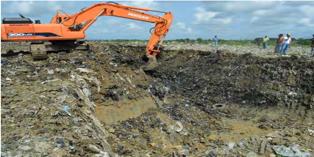
Photo 2 Excabeter in landfill
