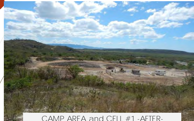
CAMP AREA and CELL #1 -AFTER-
