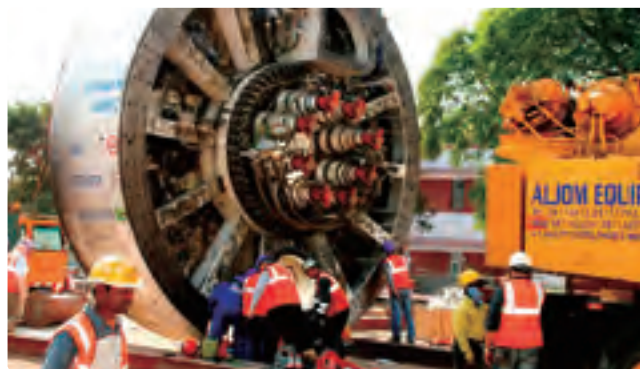
Assembling of a tunnel boring machine
