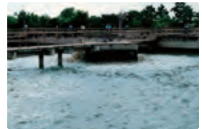
Sewerage Treatment Plant (Nagasandra)
