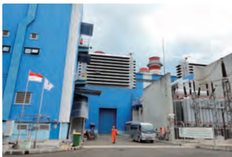
Tanjung Priok Gas Fired Power Plant
