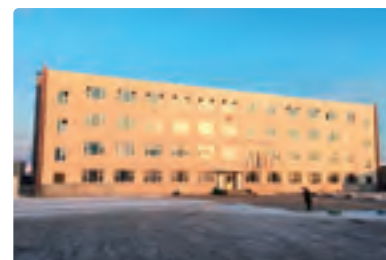
A school constructed by the project (No. 118 school)
