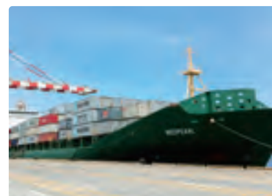
Container terminal constructed by Batangas Port Development Project
