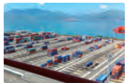
Container terminal constructed by Subic Bay Port Development Project
