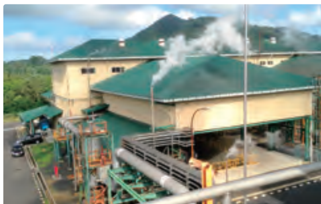
Lahendong Geothermal Power Plant
