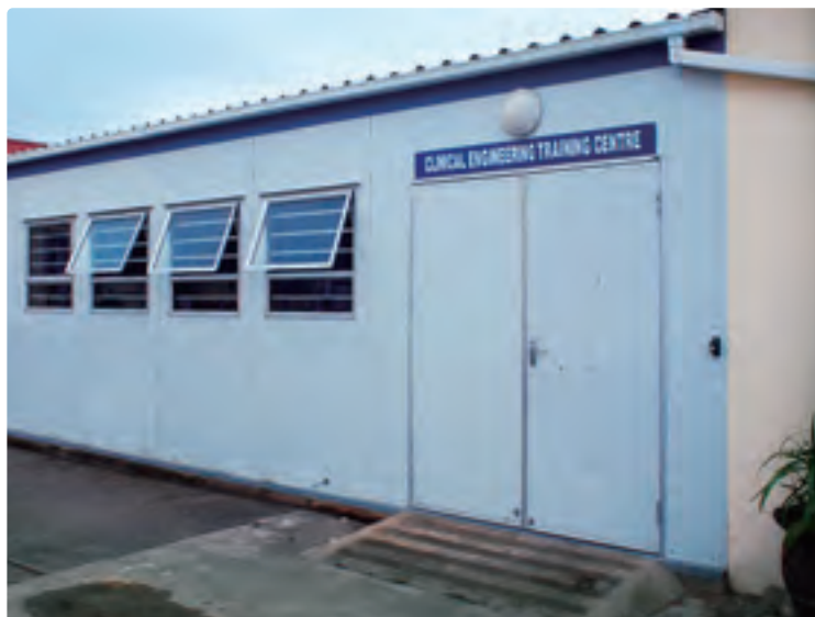
Training Center rehabilitated by the Project (Frere Hospital)
