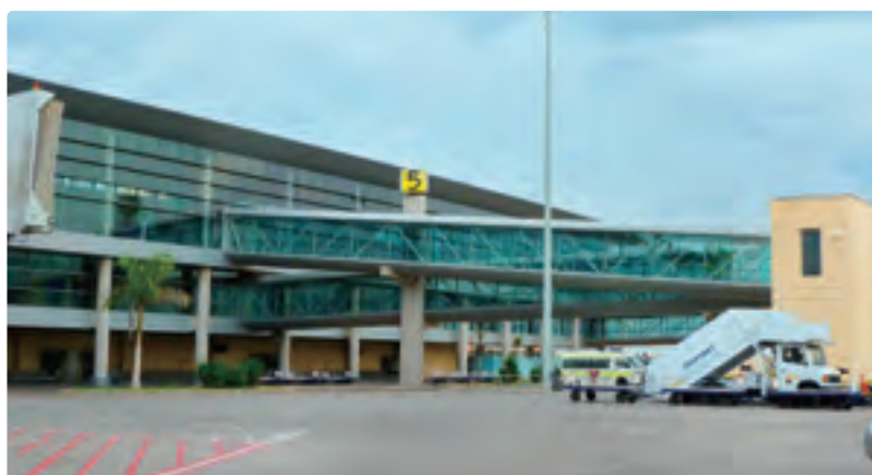
Passenger terminal constructed by the project
