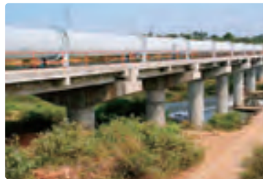
Water Transmission Line to Bangalore City
