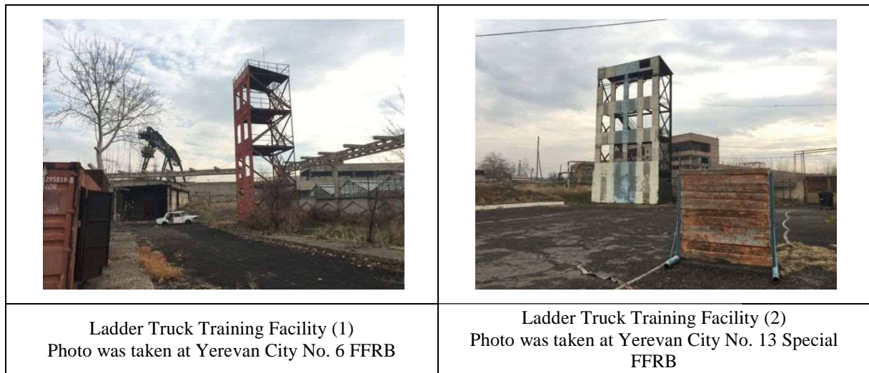
Photo 2-4 Ladder Truck Training Facility
