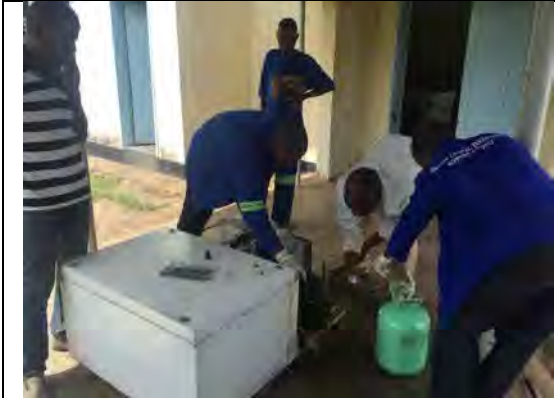
Repair work for mortuary refrigerator, Kaoma DH
