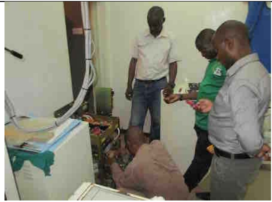
Repair work of X-ray machine, Lundazi DH
