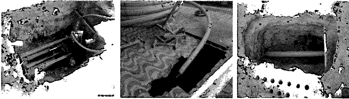
Left: Drilling Device; Center: introduction of polyethylene pipe; Right: laying completed.
