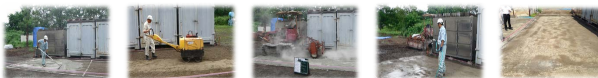
(i) Spreading out (ii) Mixing (iii) Compaction (iv) Watering (v) Completion of STEIN
