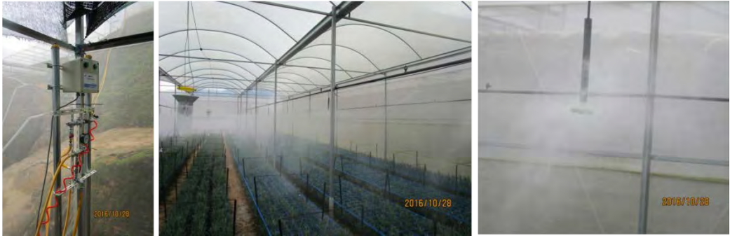
Left) Control unit, Middle) Spraying scenery, Right) Spreading mist
