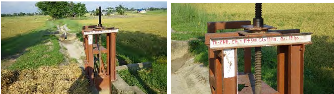
Figure 4-2-1 Sluice Gates of the Tertiary Canals in Kankai
